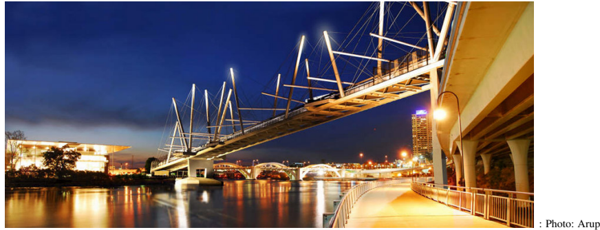
Figure 2: Kurilpa Bridge, Brisbane, Australia
