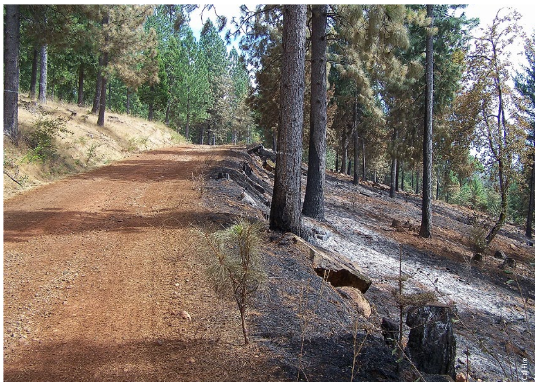
In 2006, a fire in Marysville (Yuba County) was stopped at the Oregon Ridge fuel break, which was constructed by private timber landowners as part of the Slapjack fuel reduction project.
