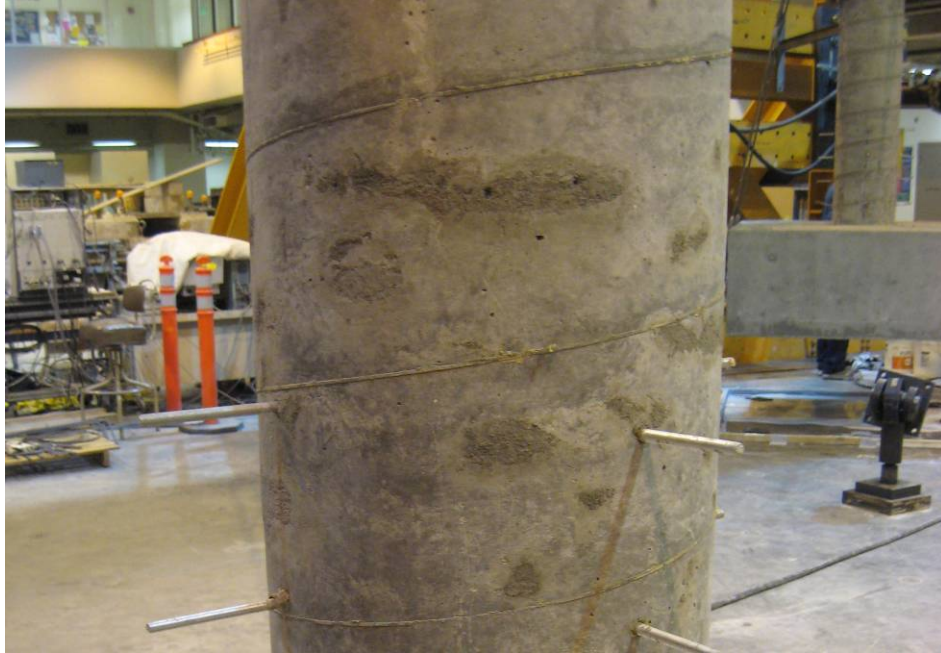
Figure B-13 Detail of S1 column after repair of cover using high-strength grout
