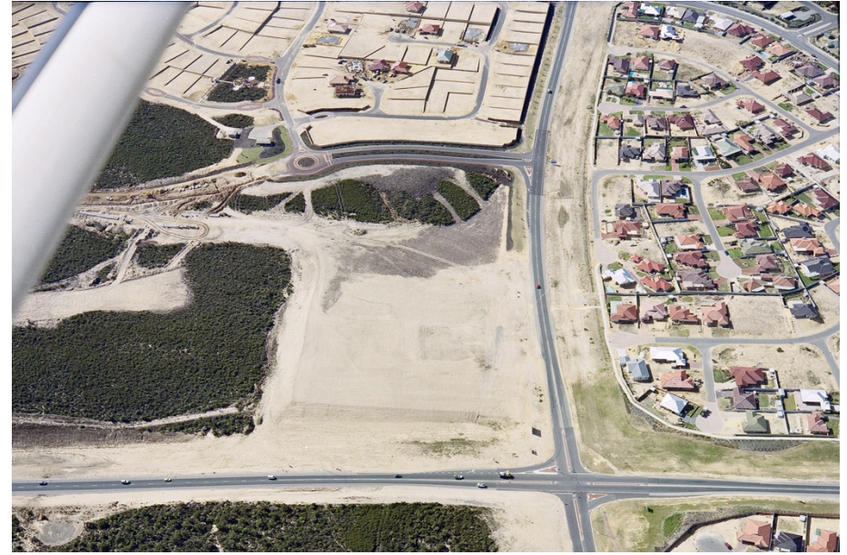
Figure 17: 1993 oblique aerial view of the development of Kinross (left background), illustrating the first extensive use of retaining walls between all lots. By comparison, the mostly developed suburb of Currambine (right middle-ground) does not include retaining walls along property boundaries (courtesy Aerial Surveys Australia, State Library of Western Australia).
