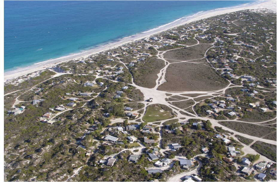
Figure 6: oblique aerial view of Wedge Island settlement (courtesy of Wedge Island Progress Association).
