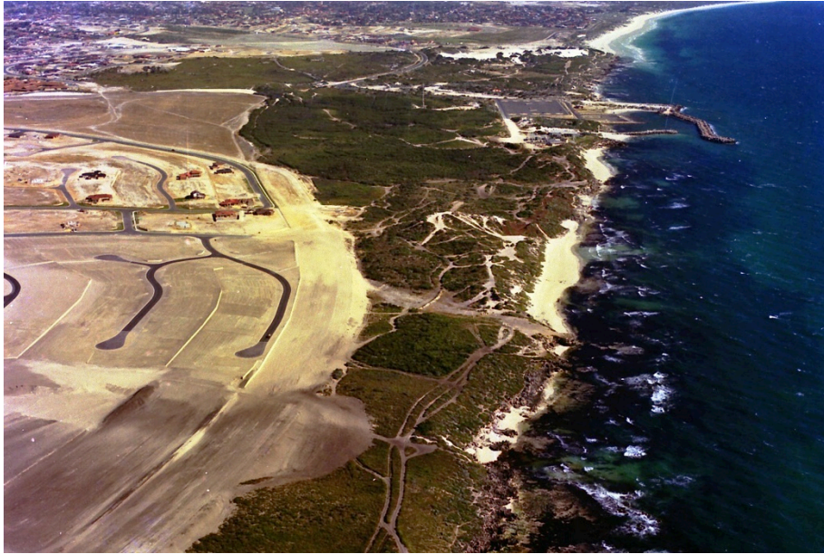
Figure 16: 1987 oblique aerial view of Ocean Reef. Retaining walls are evident behind, but not between, lots (courtesy of City of Joondalup Local History Library).
