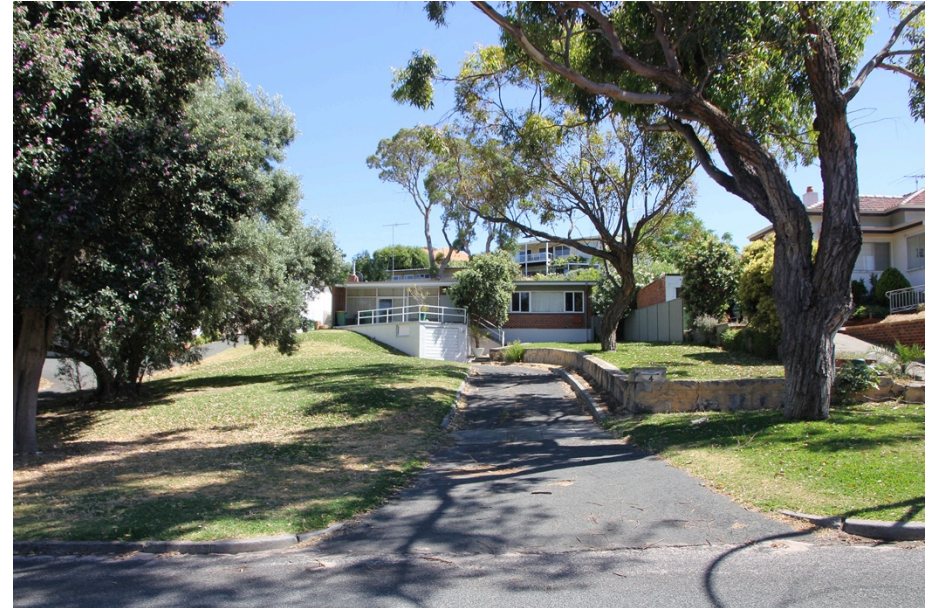
Figure 10: ground-level view of circa late 1950s City Beach house and front yard with combination of plinth, low onsite retaining walls, and embankments to negotiate level change between street and house (author 2013).
