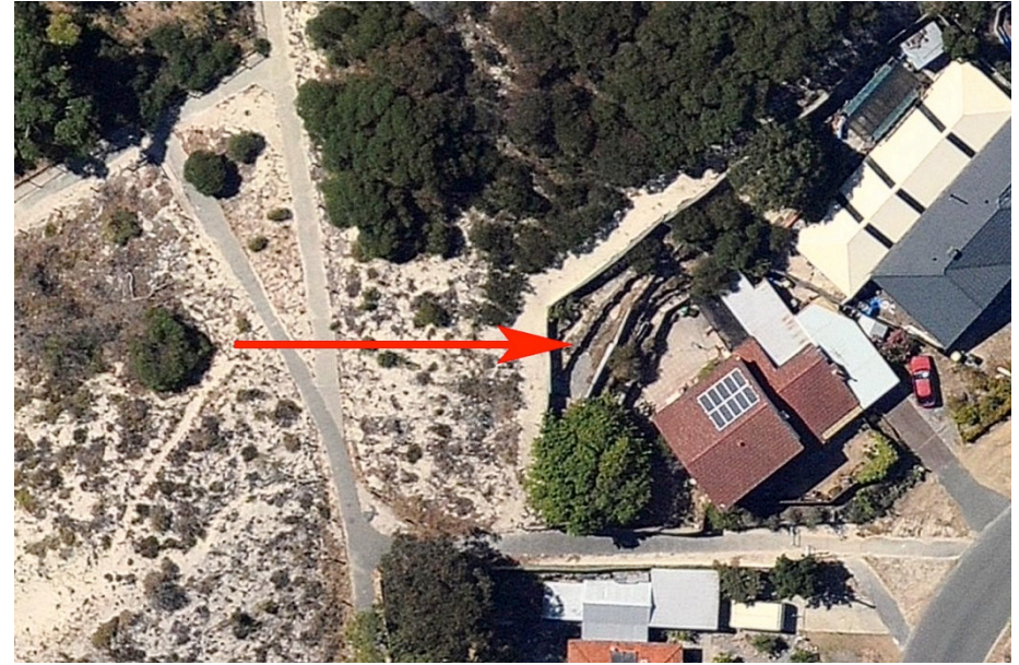
Figure 14: aerial view of back yard terracing to accommodate level outdoors entertainment area on sloping site, Kallaroo (2013).
