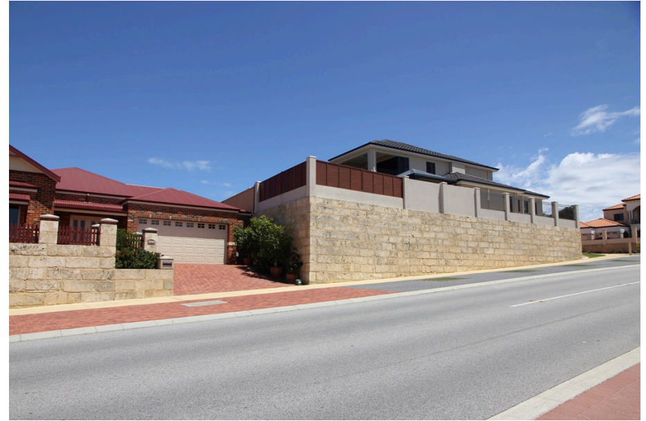
Figure 19: ground-level view of Mindarie Keys streetscape illustrating division created by 4.5m high combination retaining wall/boundary wall between adjacent lots (author 2013).
