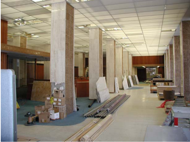
Figure A- 28: Whole Building Internal Renovations in Preparation For New Tenants
