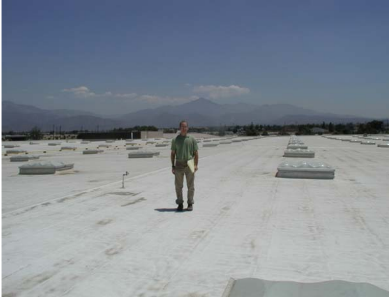
Figure A- 37: San Bernardino USPS rooftop (evaluated as potential PV site)
