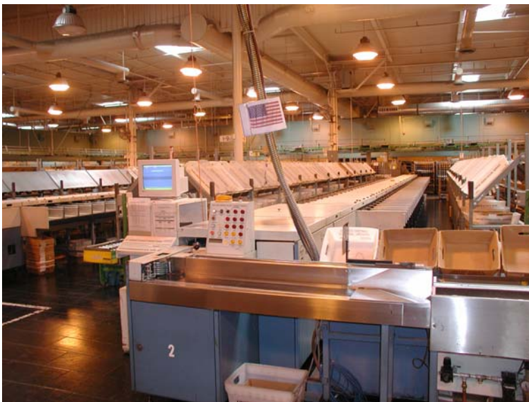
Figure A- 38: San Bernardino USPS mail handling equipment (main building area)
