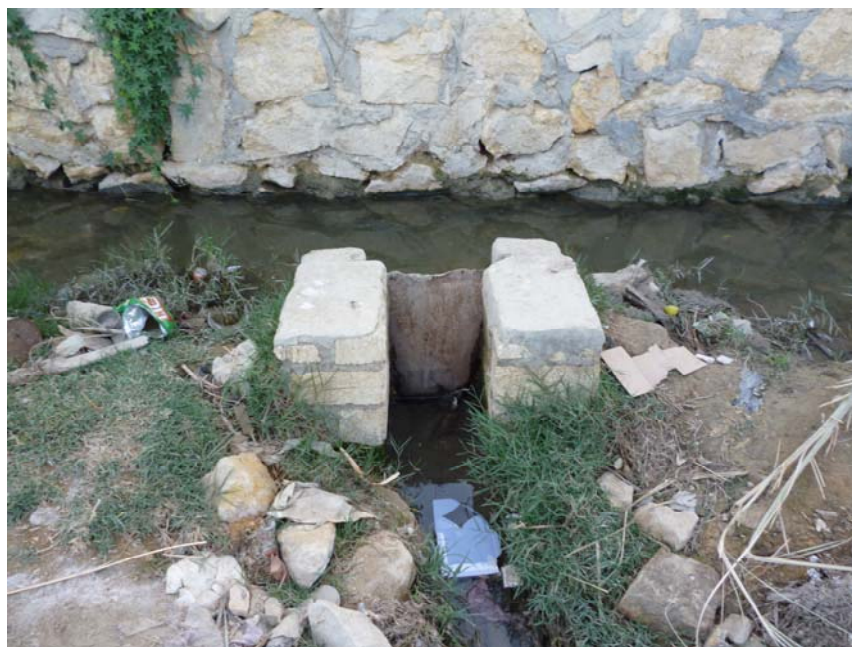
Fig. 21: A sluiceway on a branch canal in ‘Izbat Tūnsī. The simple gate is not watertight and a small amount of water constantly trickles into the field channel (conveyance loss). Photo: B. Haug, November 15, 2011.
