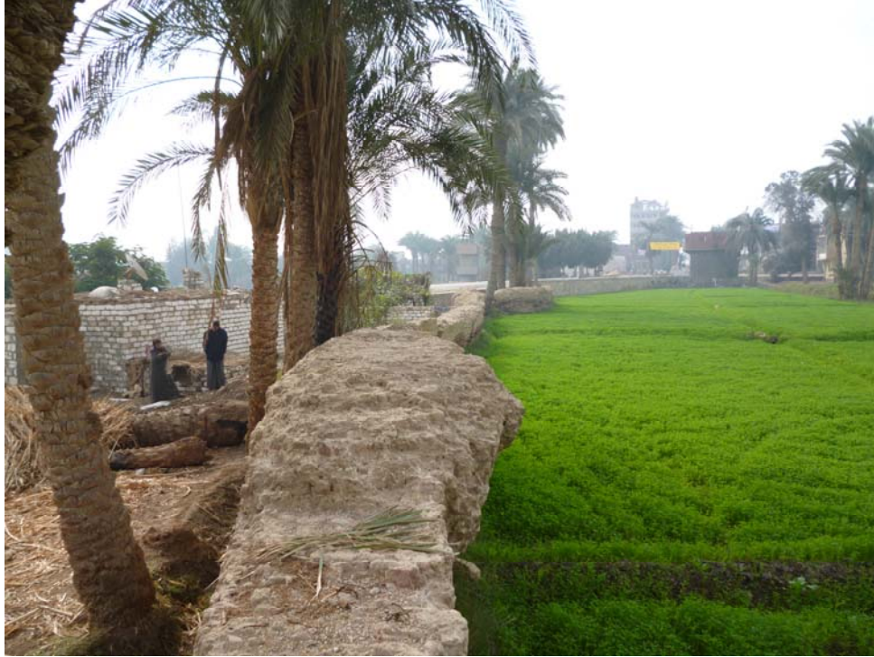
Fig. 19: A rubble core section of the dam near Itsā. In the distance the modern road has used the dam as a foundation and follows its route for a brief period. Photo: B. Haug, November 18, 2011.
