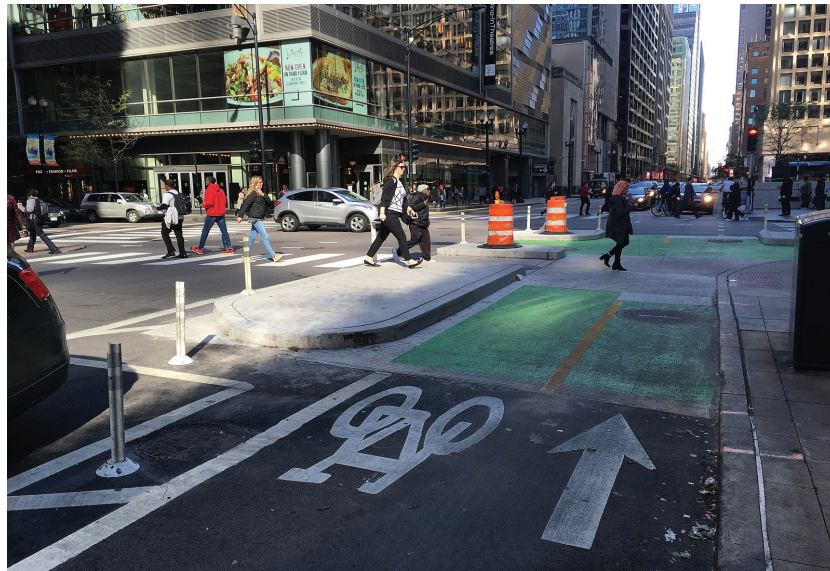
Figure 18. Corner islands for pedestrians and protected bike lane in Chicago, IL
