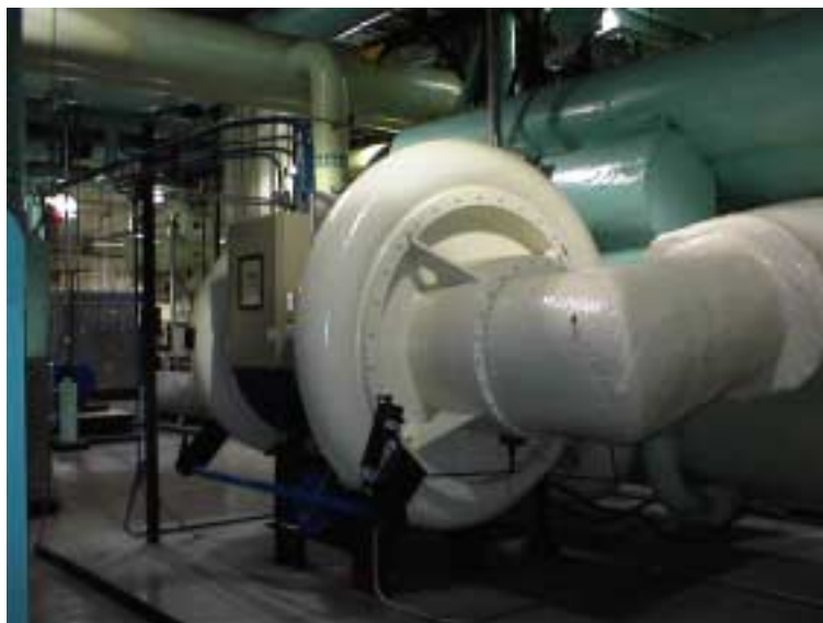
Figure 13 Centrifugal Chiller
