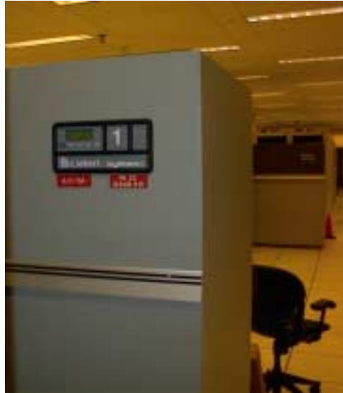
Figure 1 CRAC Unit
