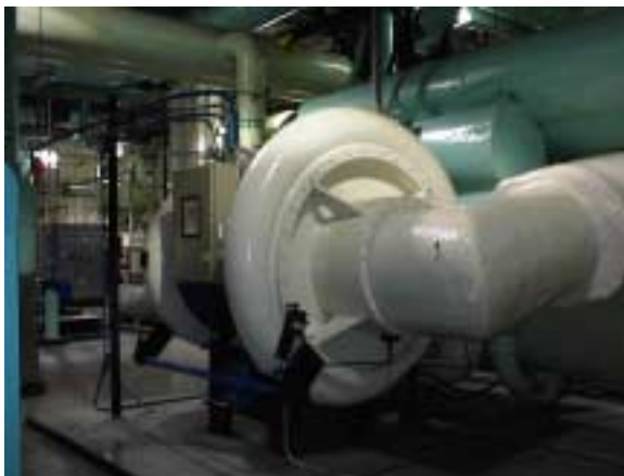
Figure 2 Centrifugal Chiller
