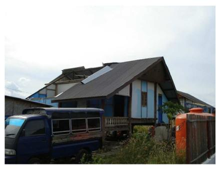
Figure 5.9: A house in Gampong Jawa with a missing roof due to strong winds less than two years after its construction had been completed
