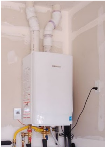
SEALED-COMBUSTION, GAS-FIRED ON-DEMAND WATER HEATER
