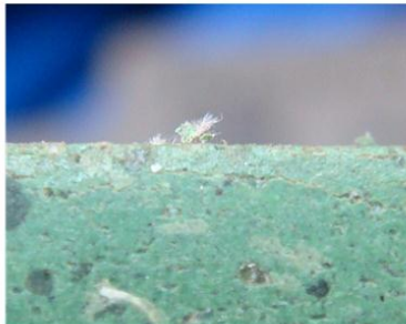
Detail of asbestos vinyl floor tile
