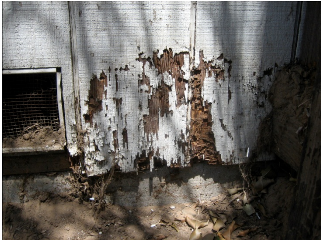
TERMITE DAMAGE
