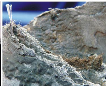
Detail of asbestos roofing felt
