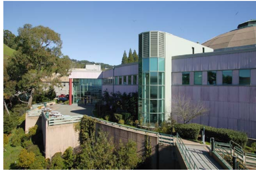
West side of the Advanced Light Source Facility
