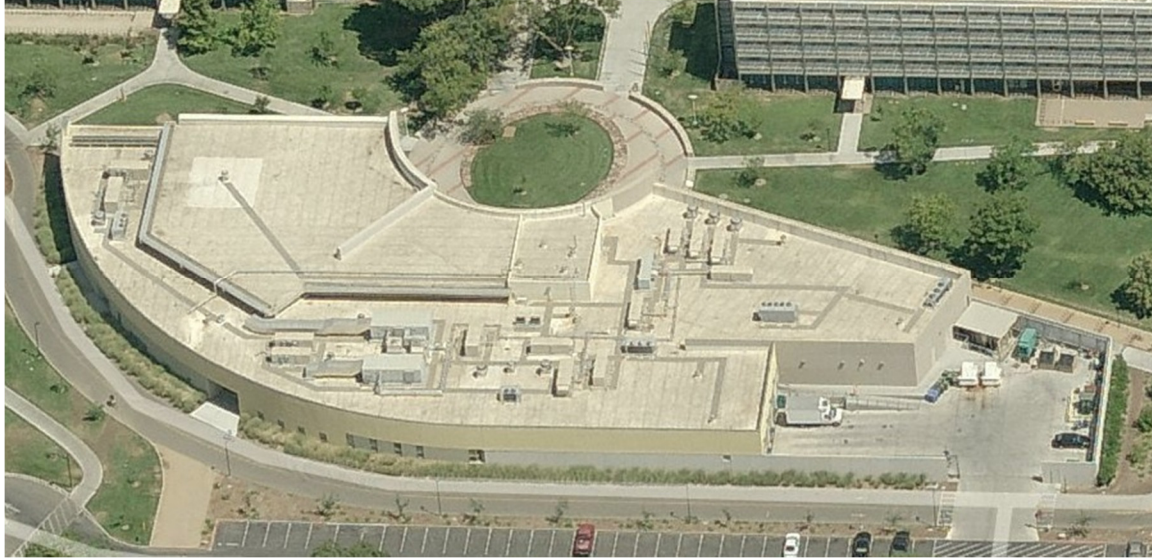
Birdseye View (from the south)
