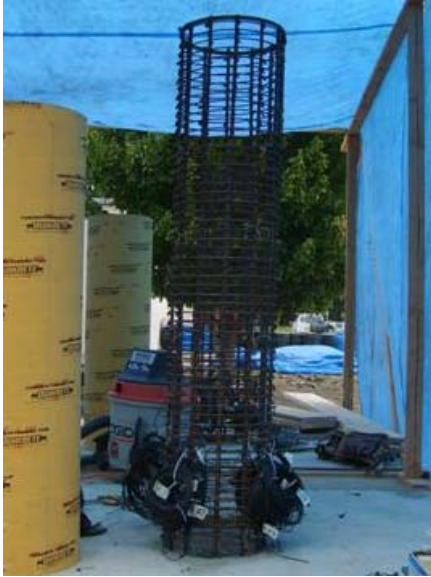
(a) After construction of the column cage
