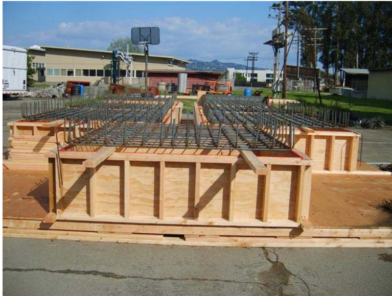
Fig. A.14 Bottom portion of the anchor block cage
