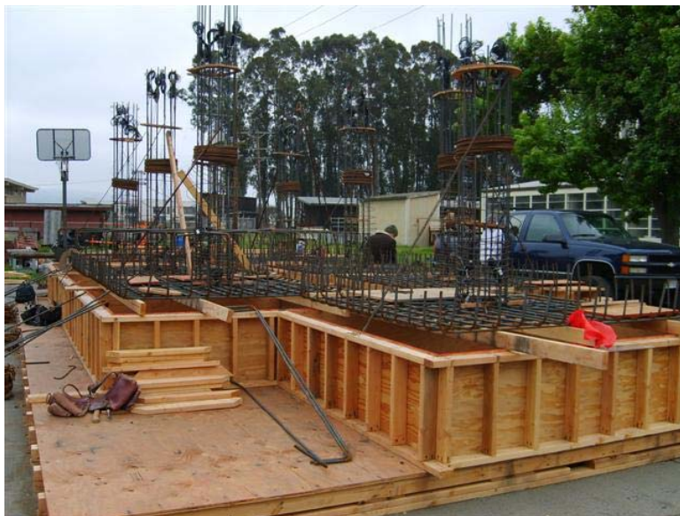
Fig. A.15 Placement of longitudinal bars
