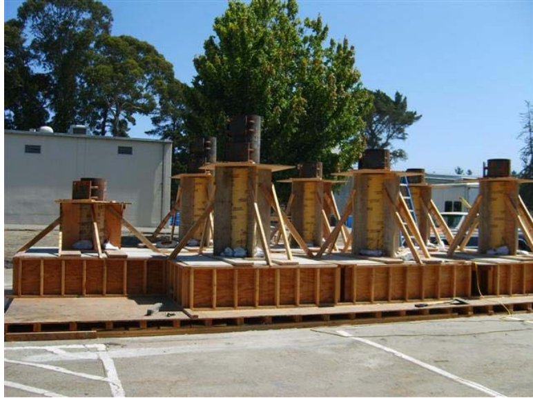
Figure A.21 Installation of steel jackets
