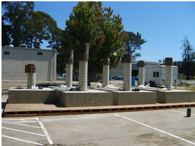
Figure A.22 After stripping the forms
