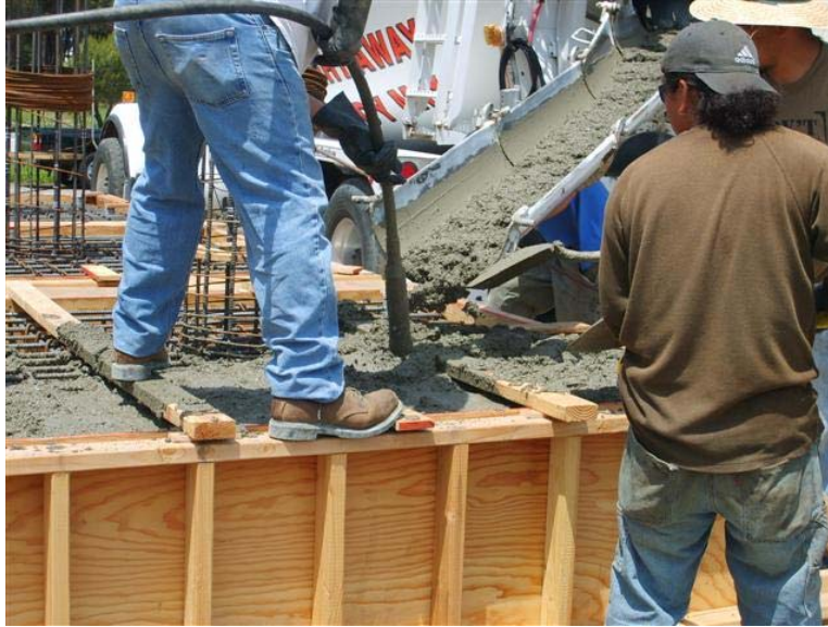
Figure A.17 Casting anchor block
