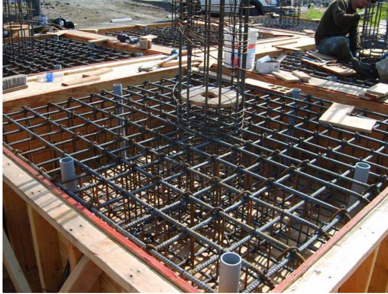
Fig. A.16 Anchor block reinforcement cage
