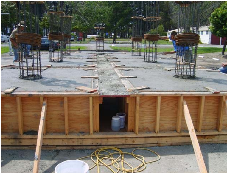
Figure A.18 After casting the anchor blocks
