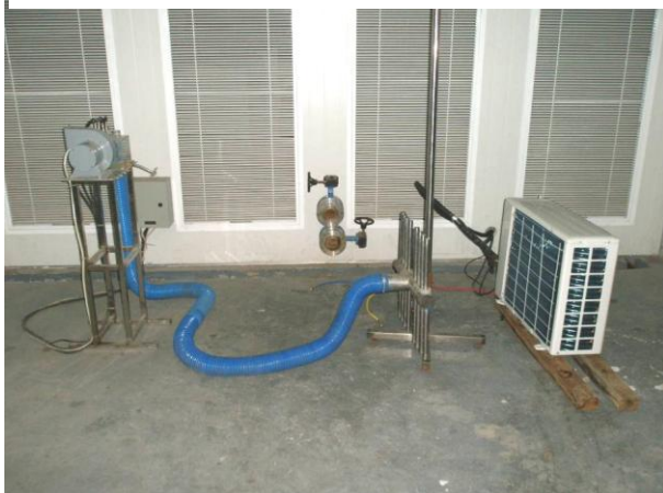
Figure 10 Air Sampling Outdoor Side at Laboratory 3
