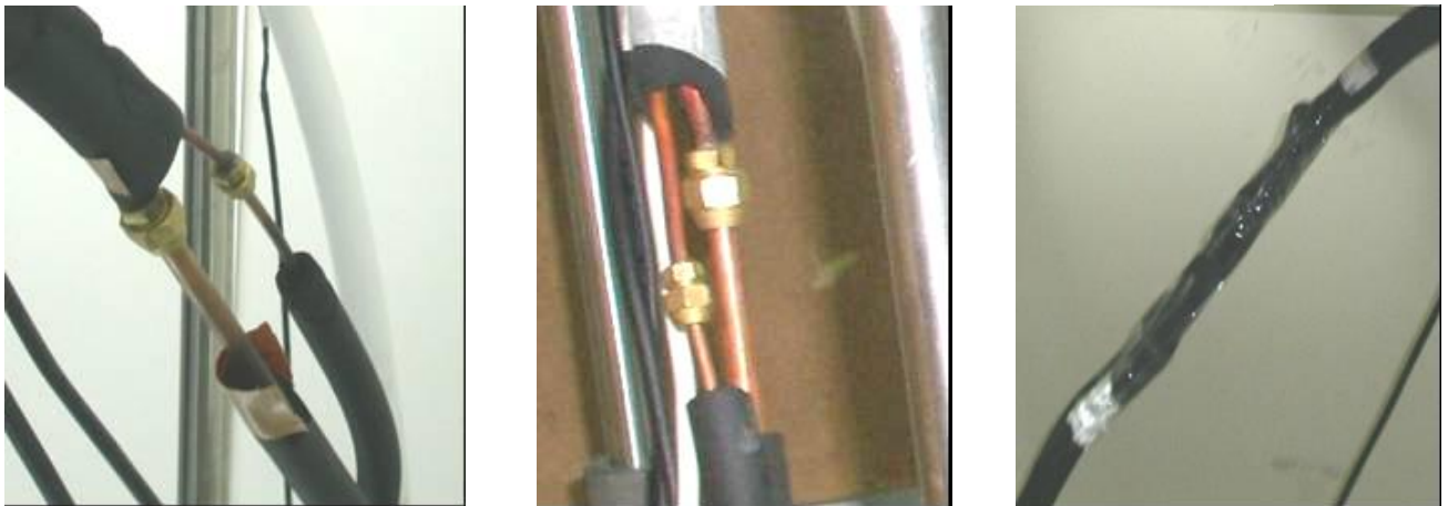
Figure 5 Refrigerant Piping Without and With Thermal Insulation
