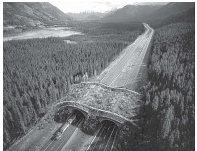
A wildlife bridge over a highway. Photo by Susan Hagood, The Humane Society of the United States
