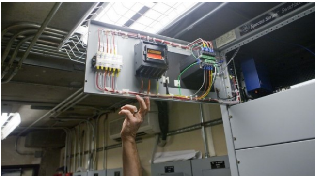
The Utilities unit provides whole-building energy monitors to document the savings generated when fume hoods are lowered. This is a smart electricity meter. All of the other meters connect into this meter for communication with our central databases.
