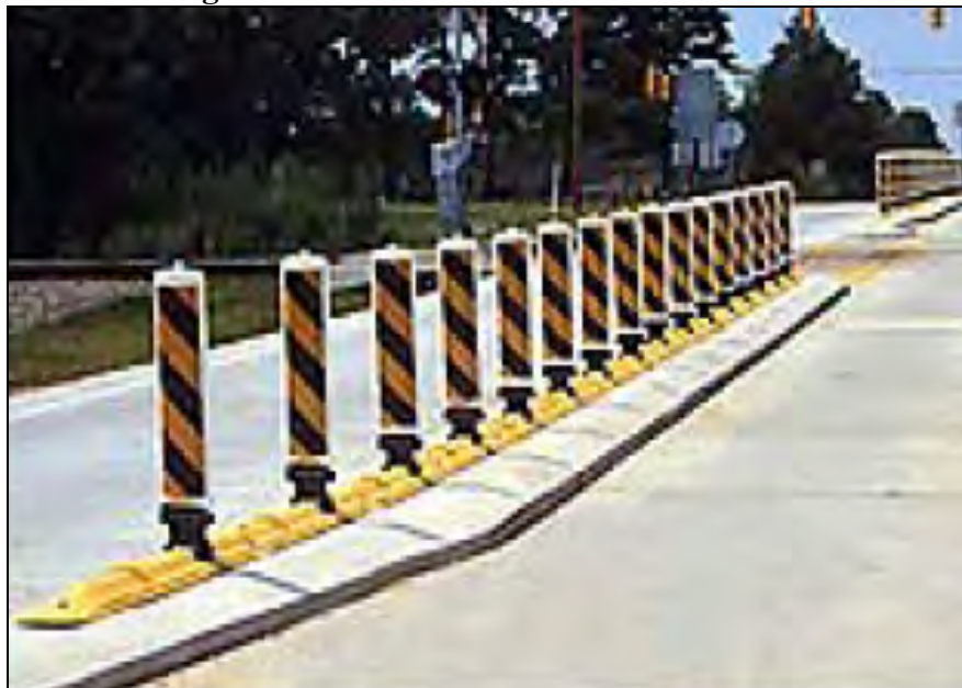
Figure 10: Island Mounted Channelization
