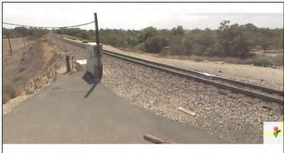
Track View 4: E of crossing, looking S
