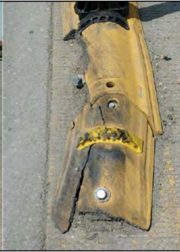
Figure 13: Flattened Curbing Caused by Trucks
