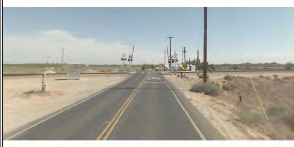
Approach View 1 Looking: East
