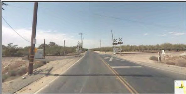
Approach View 2 Looking: West
