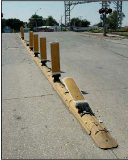
Figure 13: Flattened Curbing Caused by Trucks
