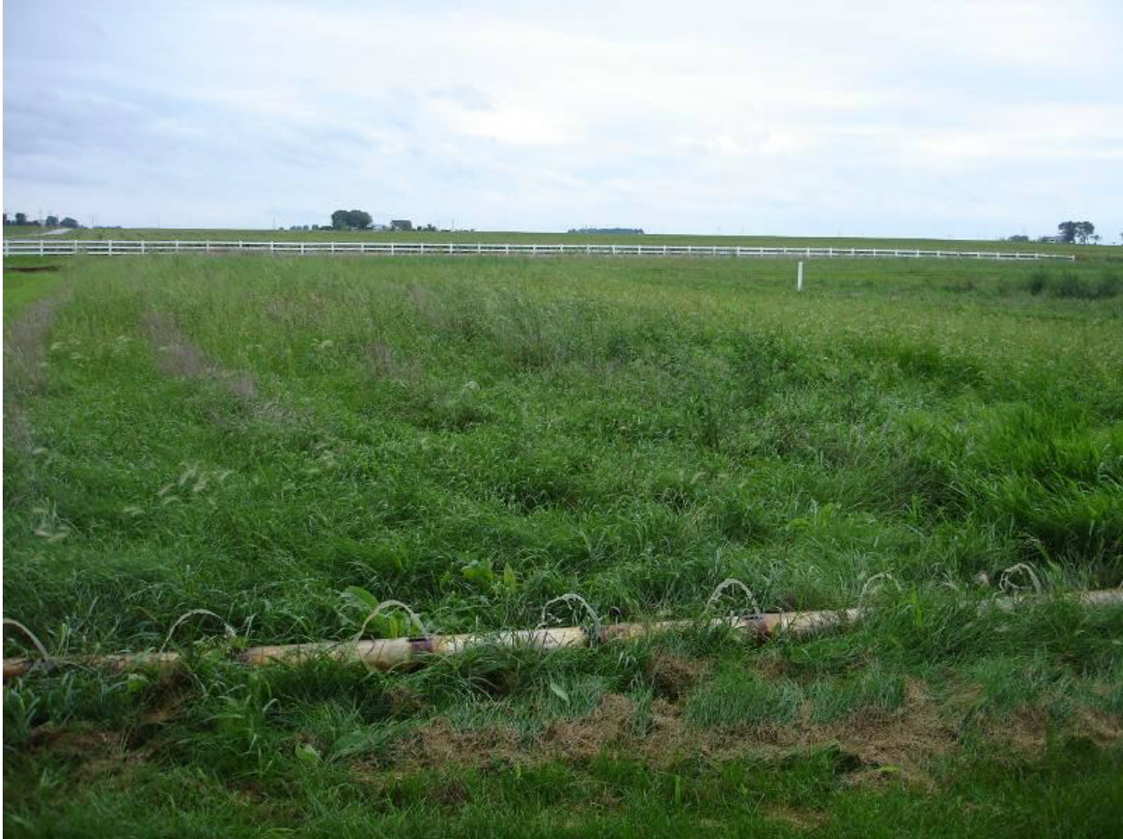
Figure 4-6. Vegetated treatment area showing effluent being applied from VIB through gated pipes.
