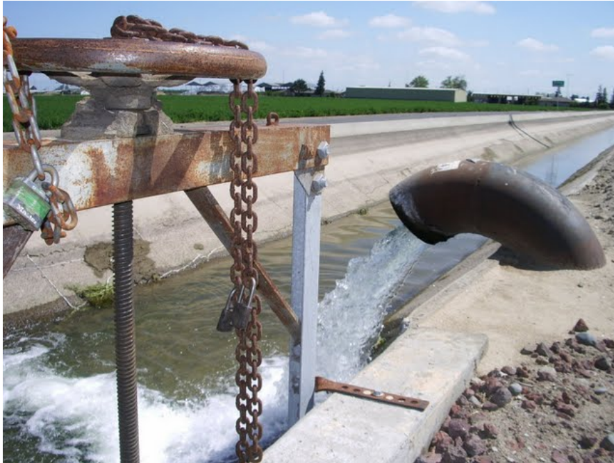
Figure 4-3. Tile drain discharging leachate drained from an area containing dairies, manure applied fields, and manure storage near Modesto, CA. (April 30, 2009)
