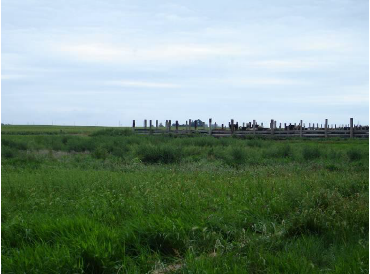
Figure 4-5. Vegetated infiltration basin receiving discharge from the solids settling basin and filtering it through the soil profile where it is collected in perforated pipes and discharged to vegetated treatment area.
