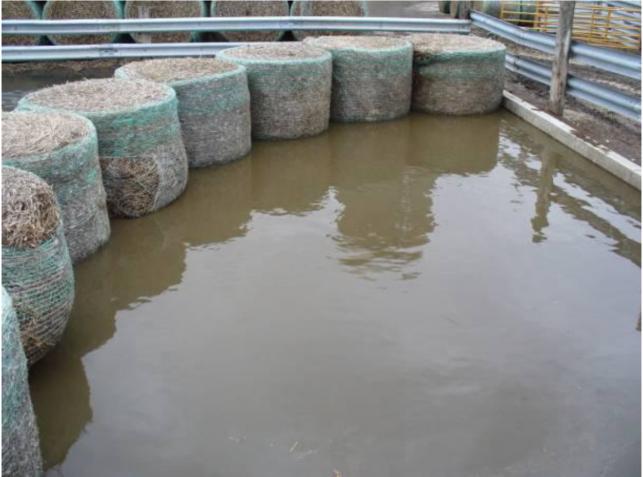
Figure 4-4. Solids settling basin collecting runoff at the Iowa feedlot.
