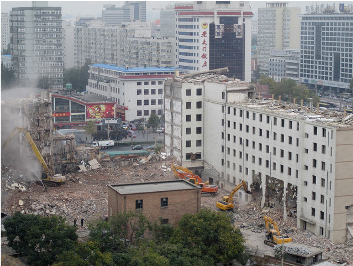
Figure 2.5 The demolition of Hademen Hotel (October 26, 2009)
