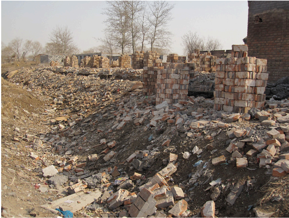
Figure 2.7 Piles of shaved bricks in Red Army Camp. (March 25, 2010)
