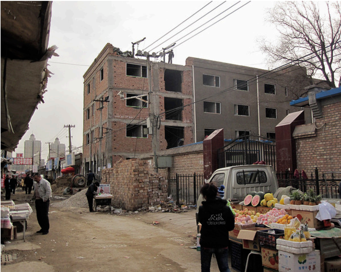
Figure 2.4 The village committee of Dongsanqi built a four-story apartment building during a tuji jianfang project. (March 25, 2010)
