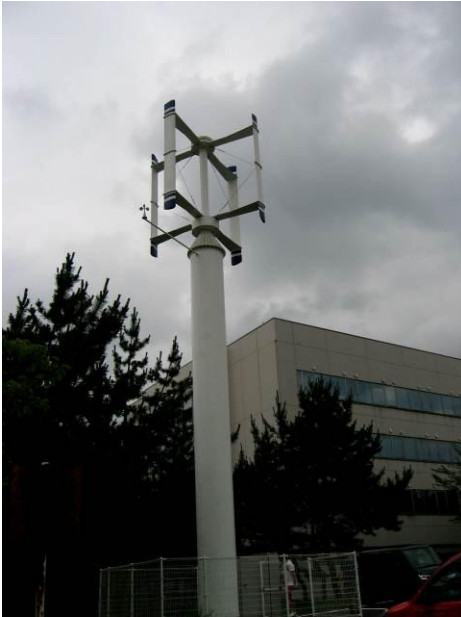
Fig. 3. Vertical axis wind turbine in the AIT DC \mu grid
