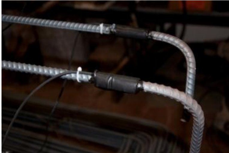
Figure A.6: Mastic Tape over Strain Gages
