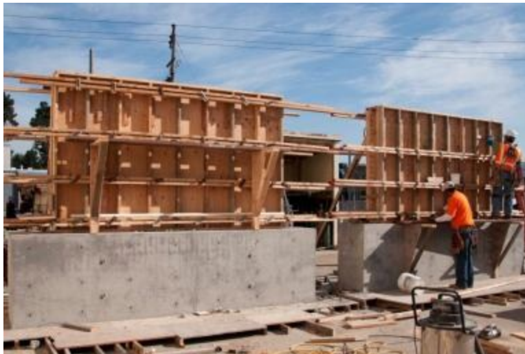
Figure A.11: Walls Formwork
