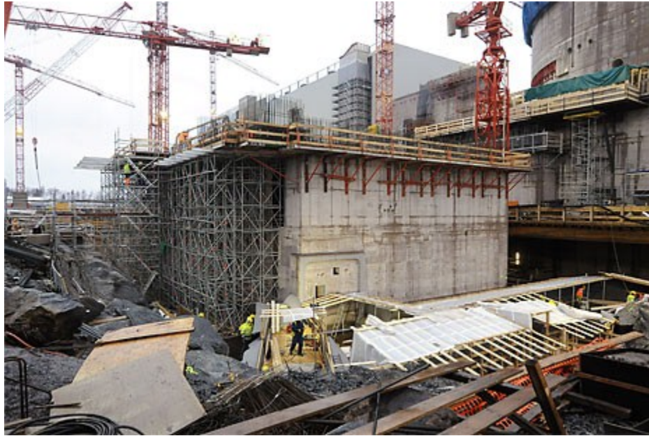
Figure 1.1 Shear Wall in Finland's Nuclear Reactor in Olkiluoto < http://www.enviro-space.com >
