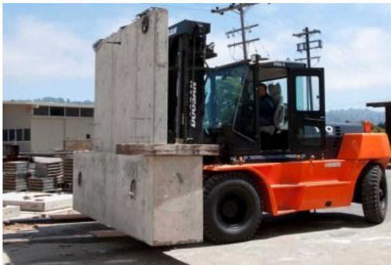
Figure A.13: Forklift Moving Wall
