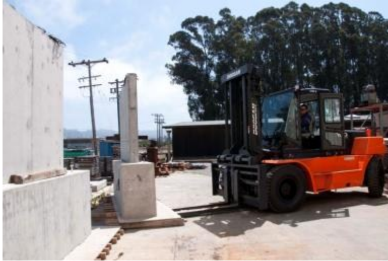
Figure A.12: Forklift Preparing to Move Wall
