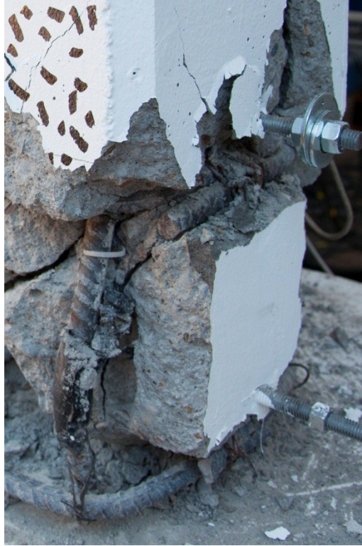
Figure 6.50: Wall 2 West Side Reinforcing Bars
