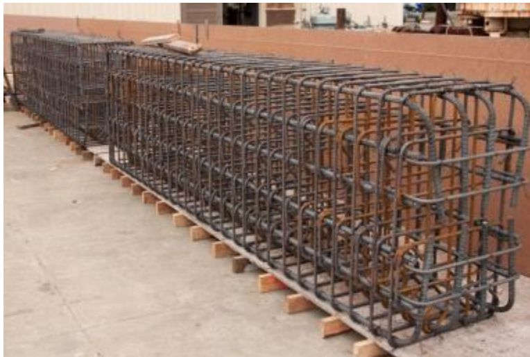
Figure A.7: Assembled Foundation Reinforcing Bar Cages
