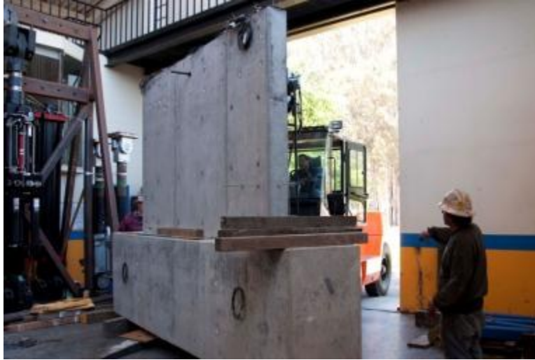
Figure A.14: Bringing the Wall Inside the Laboratory
