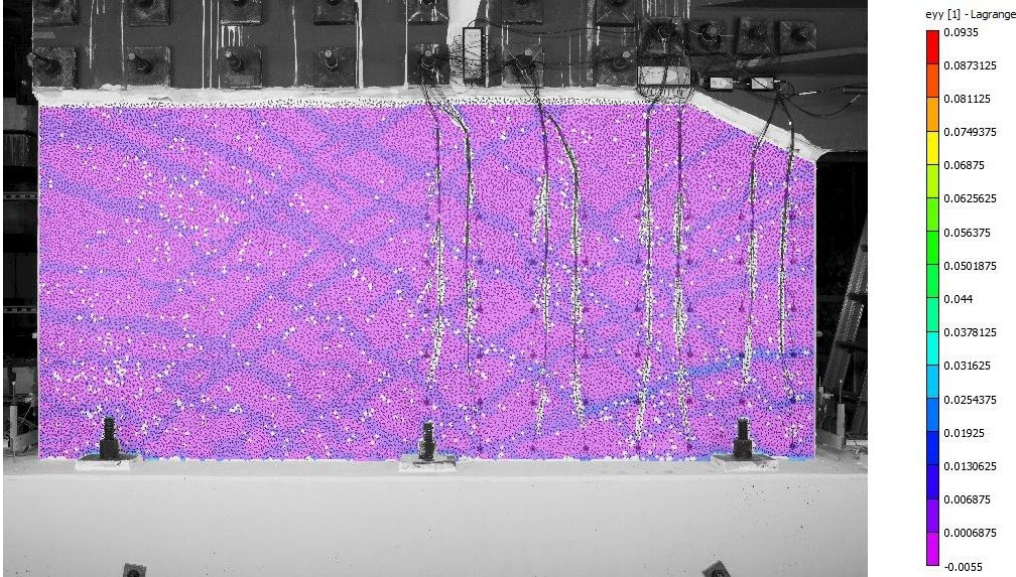
Figure 6.32: Wall 2 Shear and Flexural Cracking at Start of BDBE Motion
