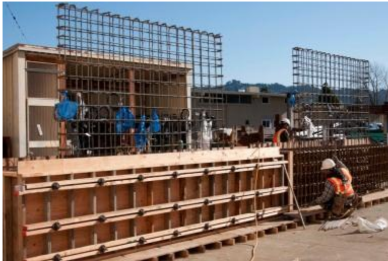
Figure A.9: Building Formwork
