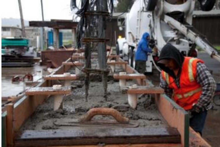
Figure A.10: Foundations Poured
