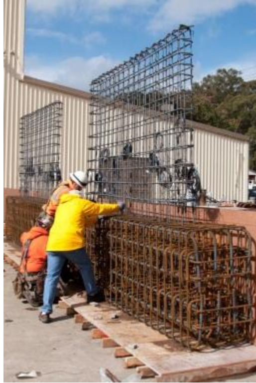
Figure A.8: Wall and Foundation Reinforcement
