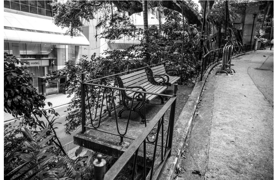
Seating ledge cantilevered over registered slope. [Karl Kullmann]
