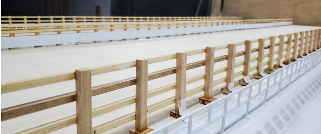
Figure 3-3-4: Close-up of railings and pavements
