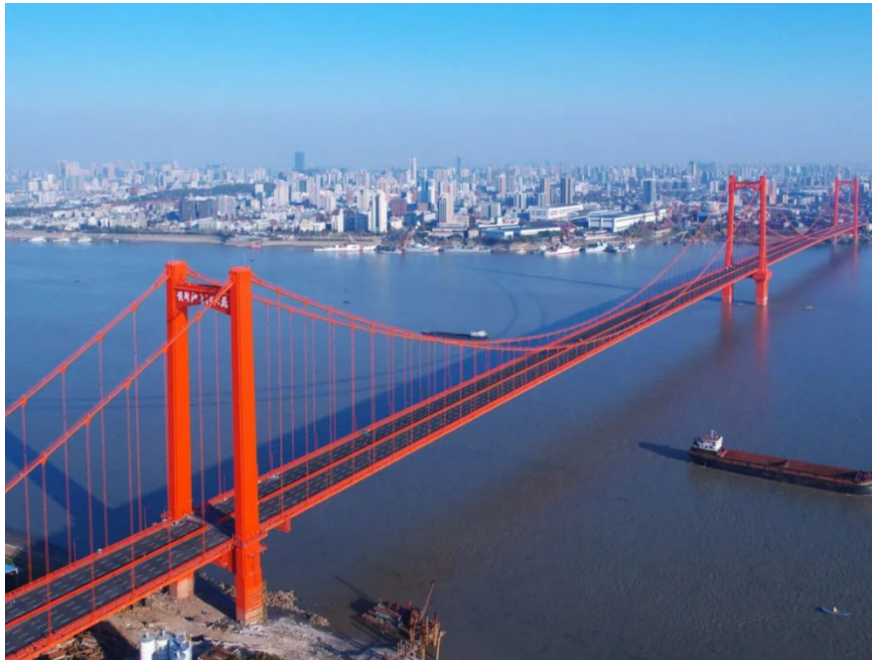
Figure 1-1-6: Yingwuzhou Yangtze River Bridge
