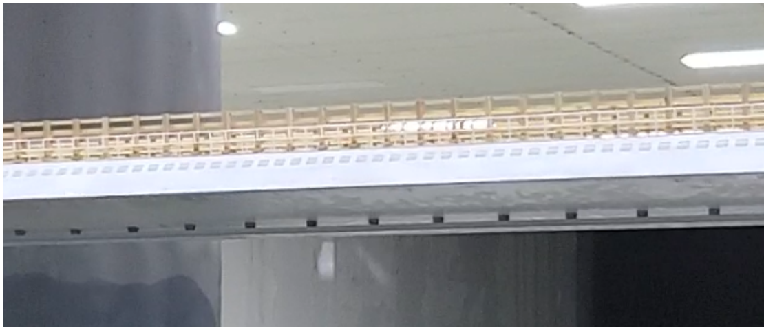
Figure 3-3-5: Maintenance tracks below the girder section
