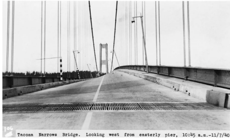
Figure 1-1-2: Tacoma narrows bridge under wind-induced vibration
