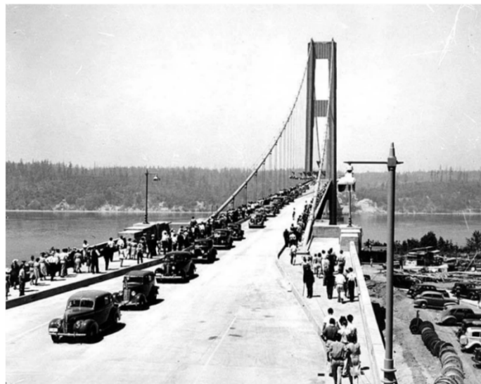
Figure 1-1-1: Tacoma Narrows Bridge on opening day ( https://www.vice.com/en/article/kb78w3/the-myth-of-galloping-gertie )
