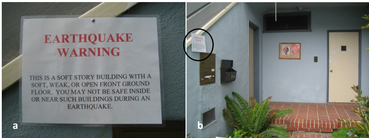
Figure 2. (a) Exemplar warning sign on the Berkeley soft-story property depicted in Figure 1, and (b) the location of that warning sign on the building.
