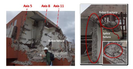
Figure 4-14. Collapsed building Torre Alto Rio
