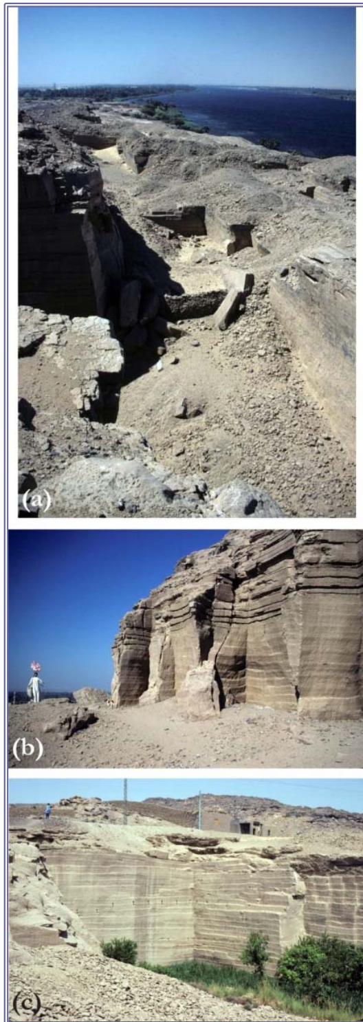
Figure 8. Examples of sandstone quarries: a) Gebel el-Silsila quarry, east bank portion (no. 11b in Table 1 and Figure 3); b) El-Mahamid quarry (no. 1 in Table 1 and Figure 3); c) Nag el-Hosh quarry (no. 8 in Table 1 and Figure 3).
