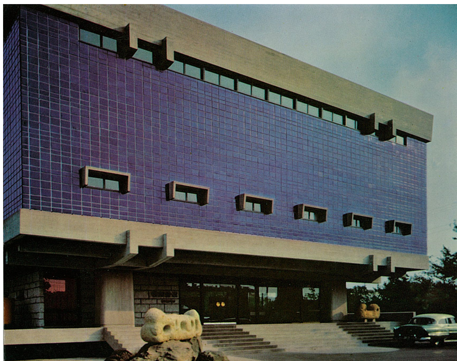
FIGURE 2.1 Image of the Sogetsu Kaikan building designed by the architect Tange Kenzo in a pamphlet announcing the new Sogetsu Art Center, 1958. Photo by Kawasumi Akio, Research Center for the Arts and Arts Administration, Keio University.
