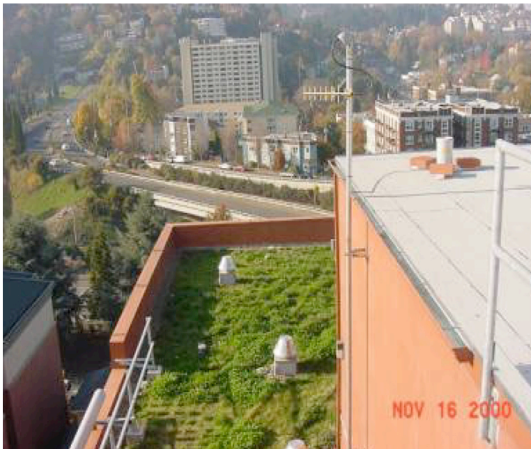
Figure 7: Hamilton Apartment — Tipping Rain gauge Station (courtesy City of Portland Bureau of Environmental Services)
