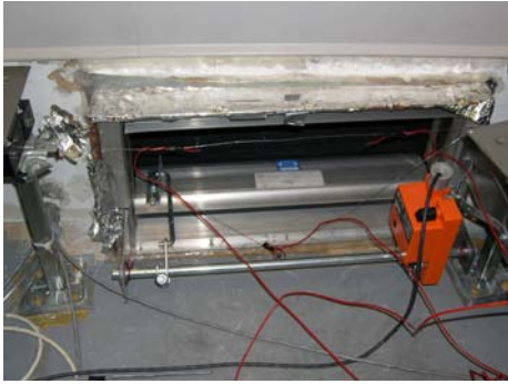
Figure 38: Supply plenum inlet control damper and sensors (3-junction average)
