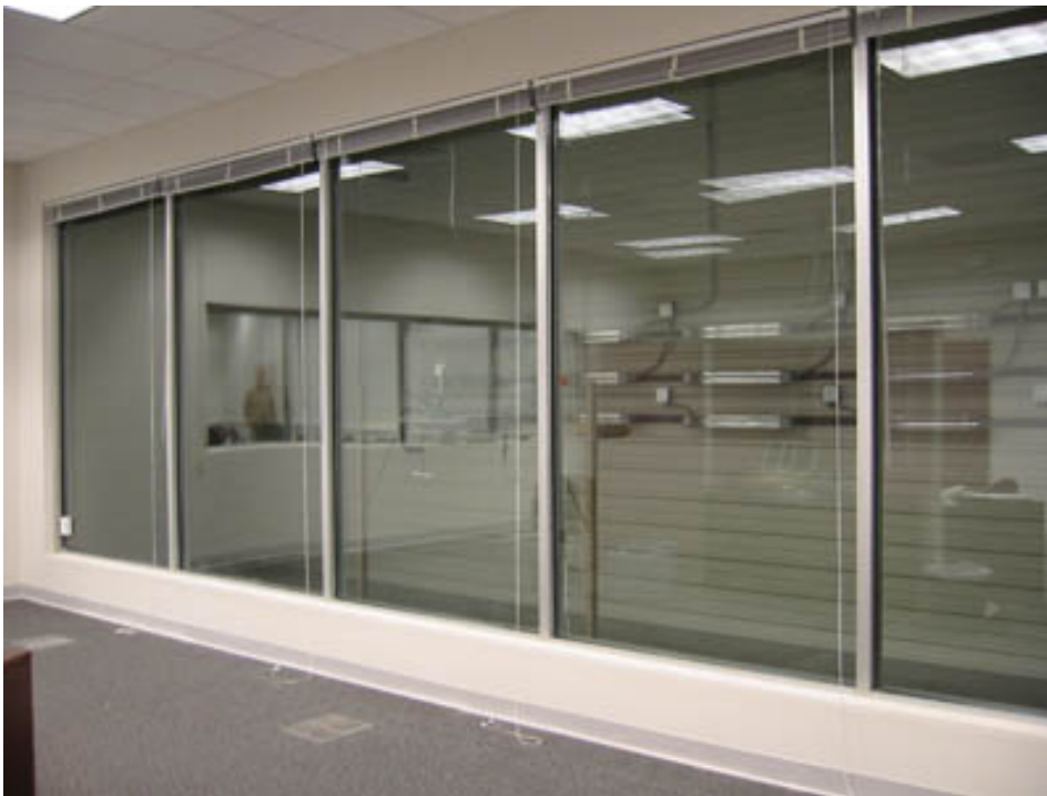
Figure 6: West wall windows, blinds open
