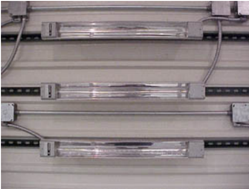
Figure 16: Quartz halogen lamps
