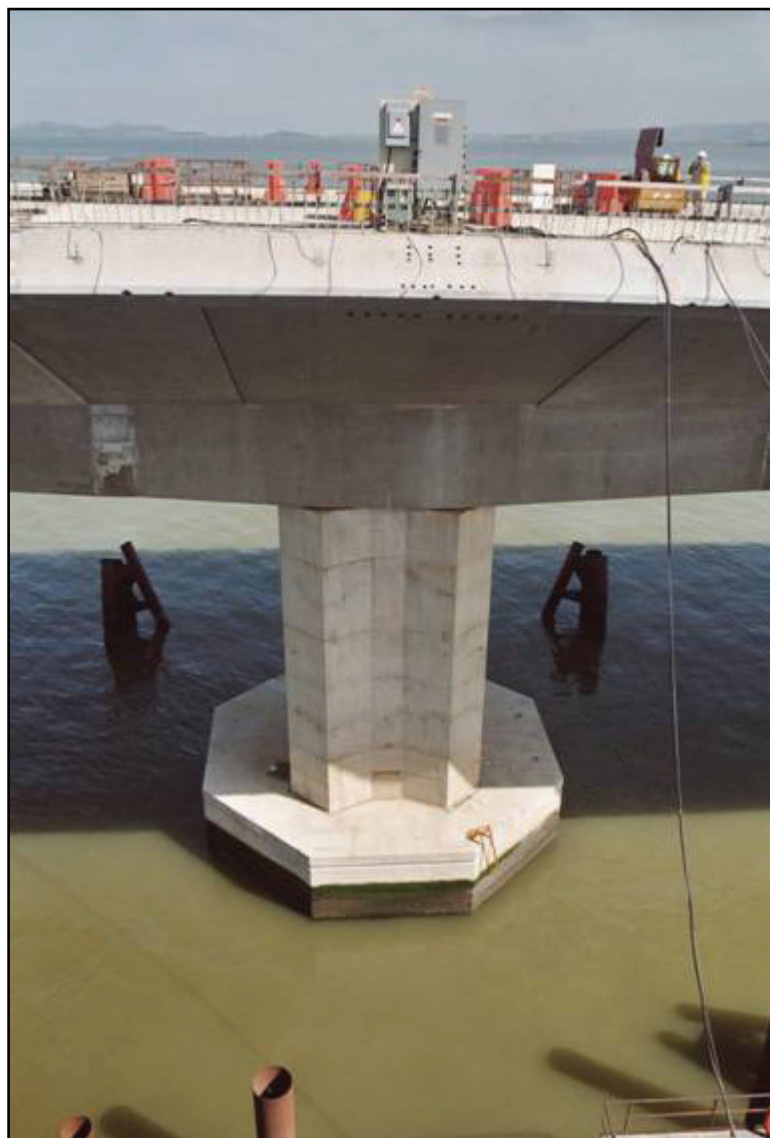
Figure A-13-42 SFOBB - Typical Pier
