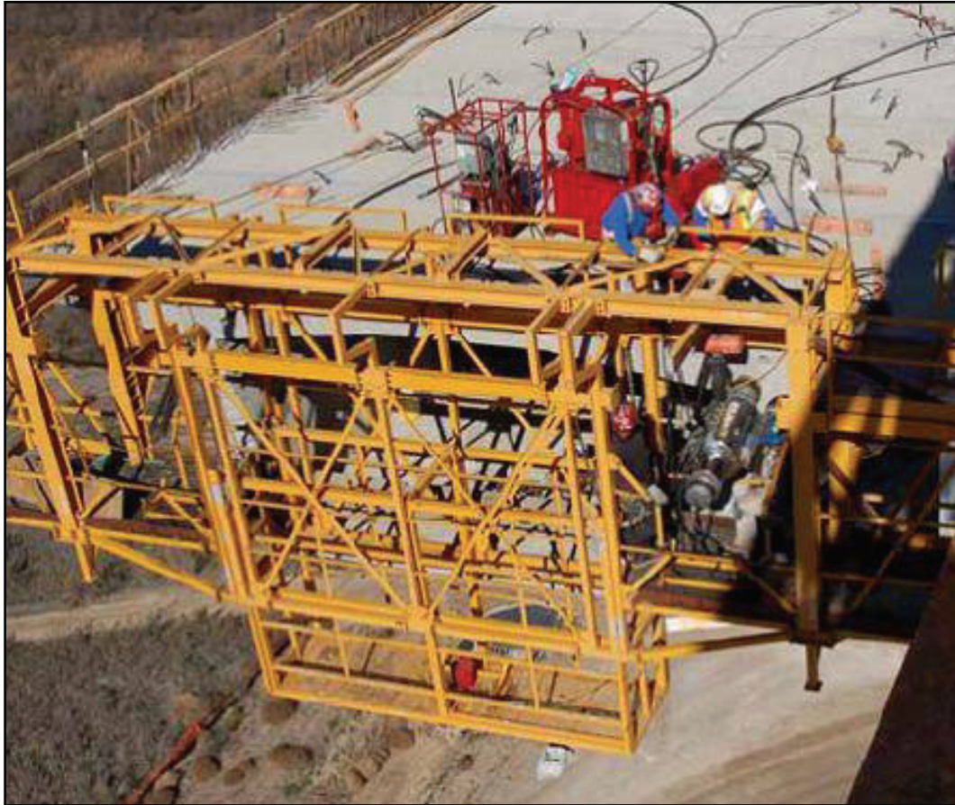
Figure A-13-51 Segment Stressing Operation (Courtesy of International Bridge Technologies)
