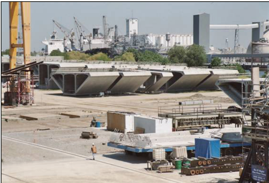
Figure A-13-38 SFOBB - Segment Storage
