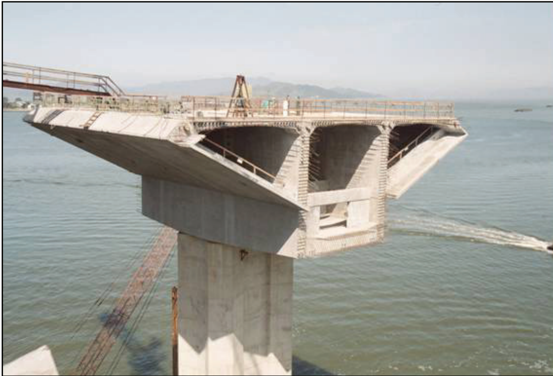
Figure A-13-40 SFOBB - Pier Table
