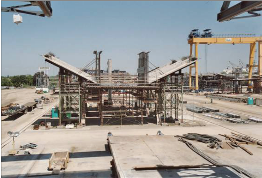
Figure A-13-37 SFOBB - Casting of Segments
