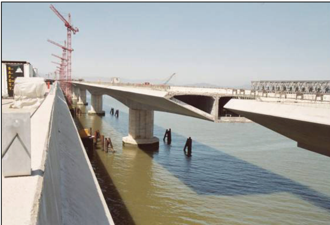
Figure A-13-41 SFOBB - Looking West
