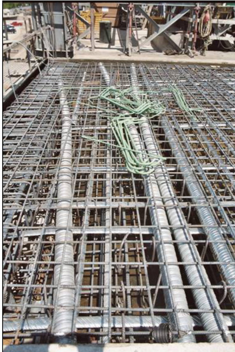
Figure A-13-36 SFOBB Deck Reinforcement and PT
