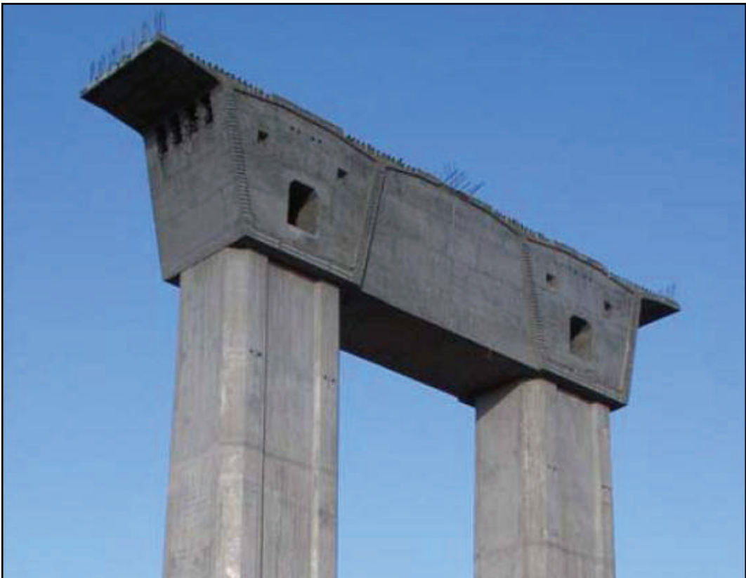
Figure A-13-46 Otay River Bridge - CIP Pier Table (Courtesy of International Bridge Technologies)
