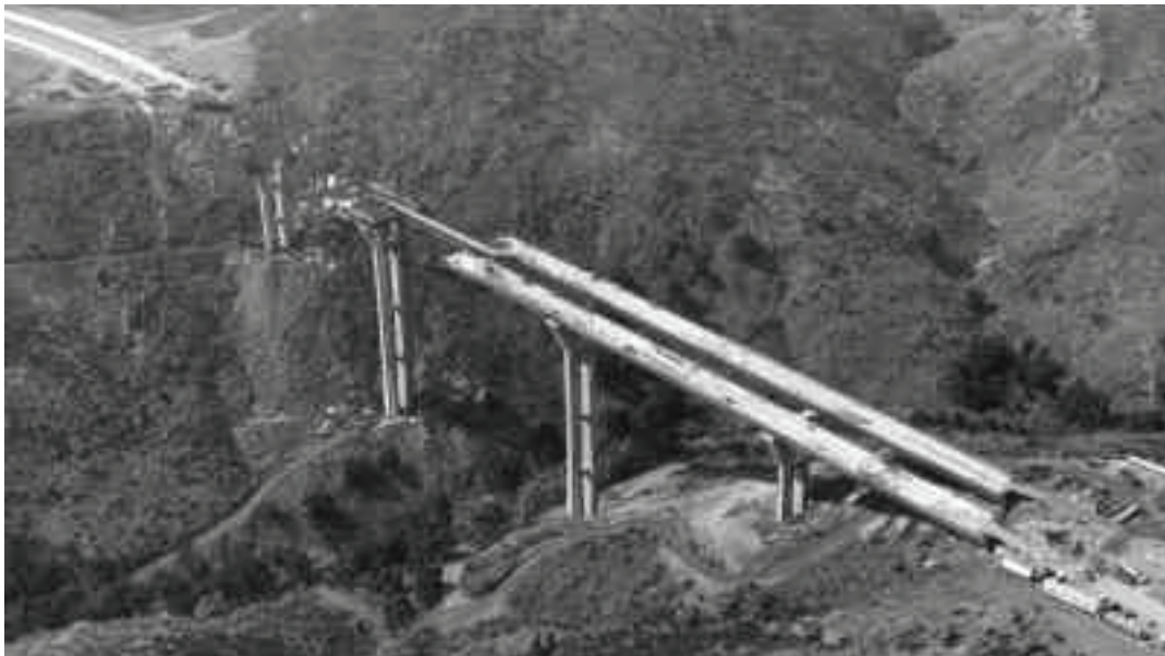
Figure 2-13 Pine River Bridge, San Diego, CA - The First Cast-in-Place Segmental Bridge in the United States (Opened to Traffic 1974)
