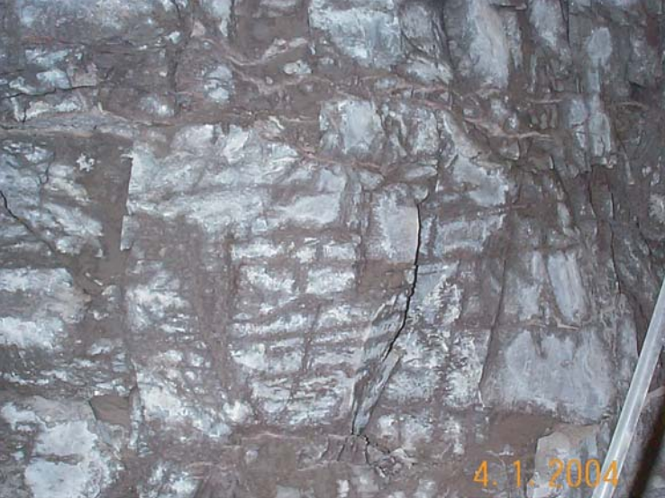
Figure 10. Water emerging along a network of fractures along back wall of Niche 3. The tube in the lower right hand corner had an outer diameter of 1 cm. This photograph shows that flow in this fractured rock is through a network of fractures which is largely made up of fractures which are less than 1m in length.
