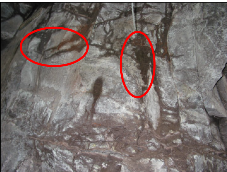
Figure 8. Development of lateral flow along the back wall of Niche 3 over a period of 24 hours. This wetting likely occurred as water was diverted from the ceiling migrated through the formation close to the walls. Circles indicate the location of changes.
