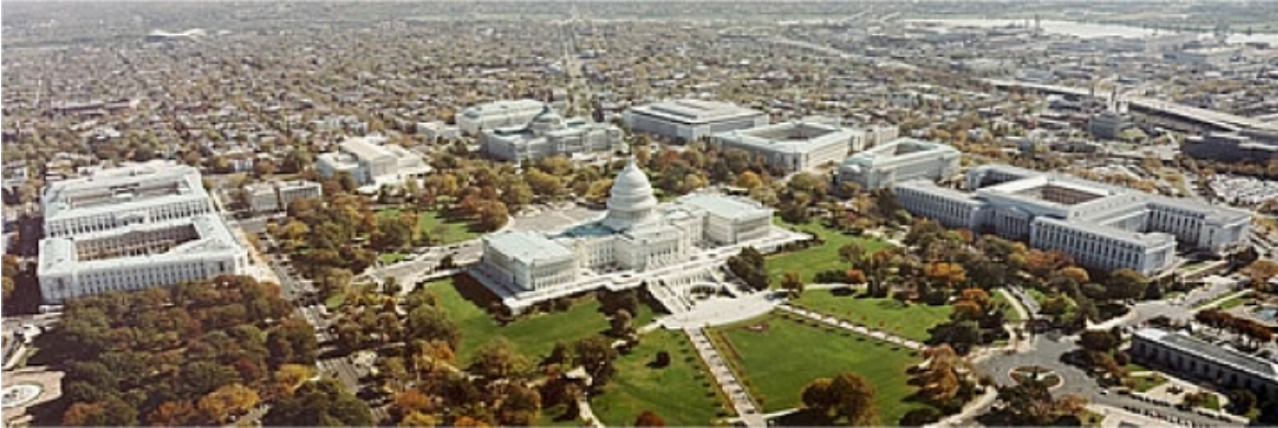
Figure 1. Aerial view of the U.S. Capitol buildings.
