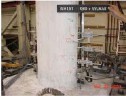
Figure 2.1- Damage state DS-1, flexural cracks.
