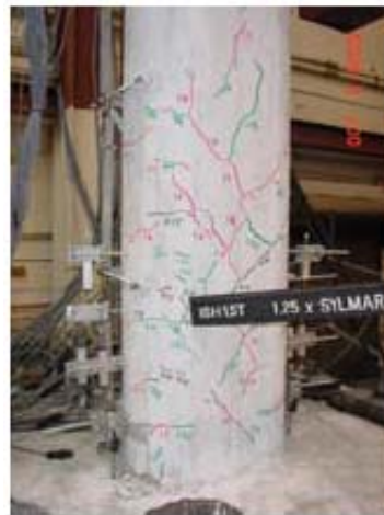
Figure 2.2- Damage state DS-2, spalling and shear cracks.
