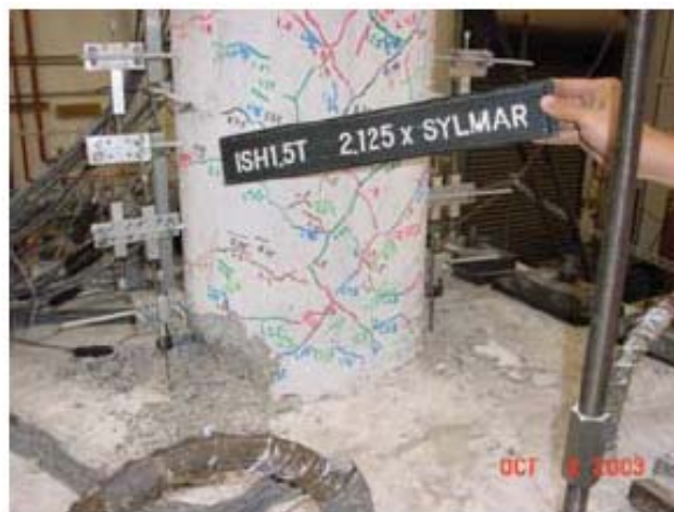
Figure 2.4- Damage state DS-4, spiral and longitudinal reinforcing bars visible.
