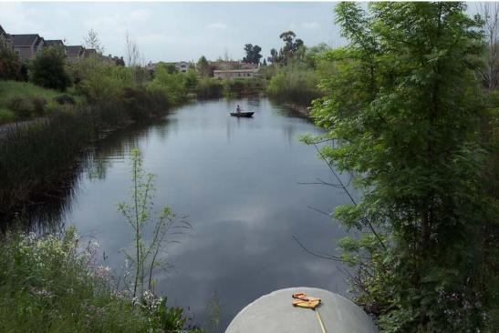
Photo 1. Photo taken of Pond A from the north end with main pipe inflow (bottom). We had to boat around the pond to survey the dimensions and take water chemistry readings. The thin ring of tule vegetation around the pond edge is growing mostly on an engineered "safety ledge".
