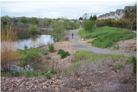
Photo 5. Pond C in the foreground surrounded by housing. The lower road is designed to allow vehicle access to the ponds for maintenance. Note that the entire area can handle much larger inflow during large storm events
