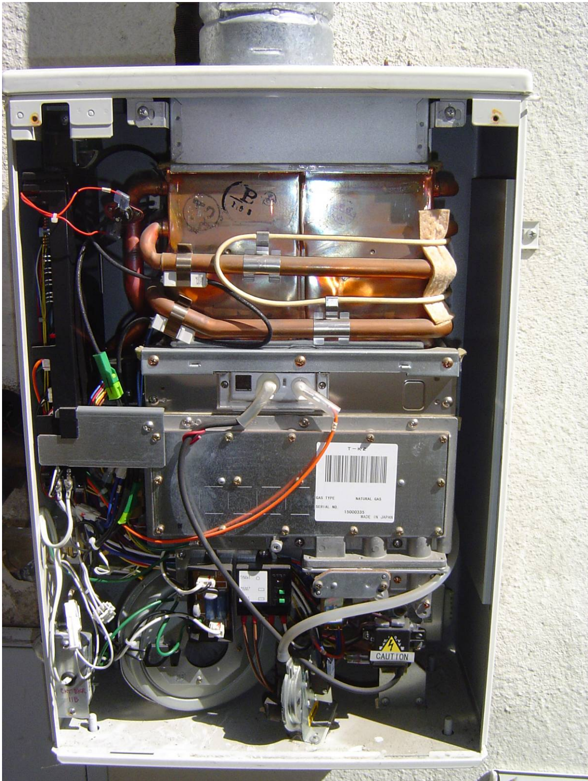
Figure 1 Takagi tankless water heater with front cover removed.
