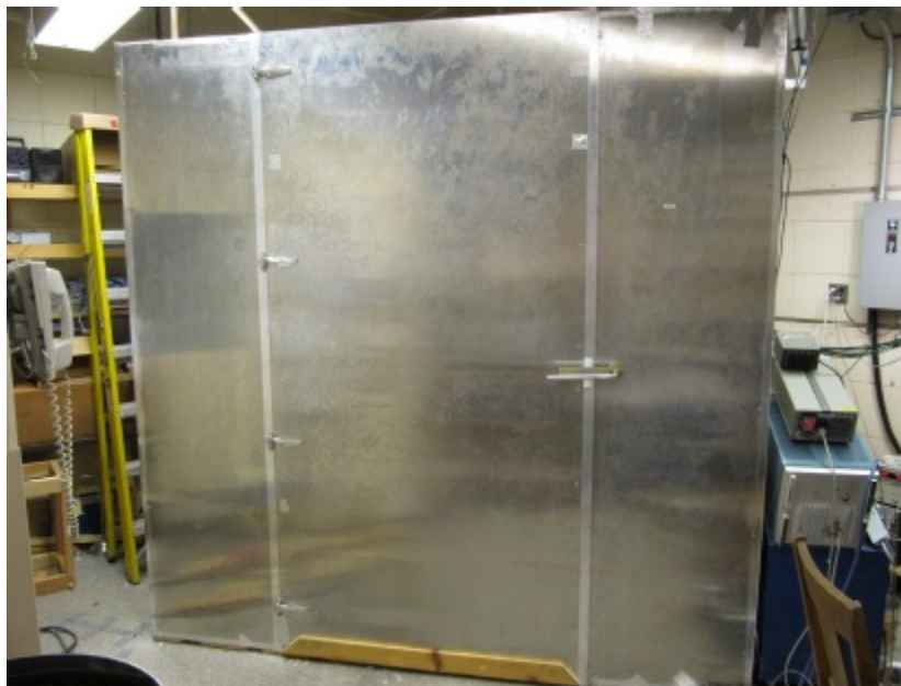
Figure 5.6. Photograph of the new aluminum shielded room.
