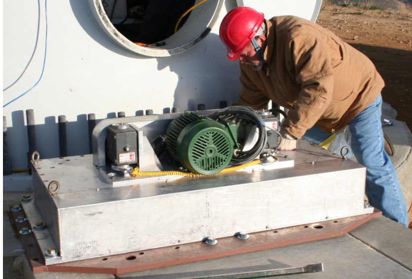
Figure 2.6: Shaker being mounted onto the wind turbine base. (Source: Prowell, 2010a)
