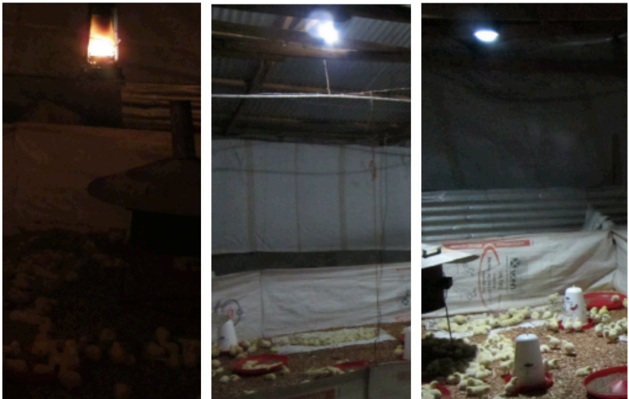
Photos: left to right. Chicken houses under illumination from kerosene lanterns, fluorescent lamps and LED lamps.
