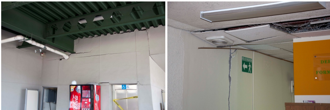
Figure 1.13 2010 El Mayor - Cucapah (Baja California) Earthquake ( M_w = 7.2 ): nonstructural damage at the Facultad de Ciencias Administrativas of UABC Mexicali: (a) PW damage and (b) PW, suspended ceiling and hvac system damage.
