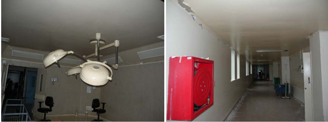
Figure 1.12 2010 Maule (Chile) Earthquake ( M_w = 8.8 ): PW wall damage from Hospital Clinica Herminda Martin, Chillán, Chile: (a) PW cracks in surgical room and (b) widespread PW cracks within a hallway. (Photos from: G. Mosqueda)
