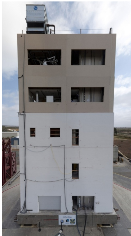
Figure 1.3 Elevation view of the south side of the five-story building test (BNCS) conducted at the University of California, San Diego. ( http://bncs.ucsd.edu )
