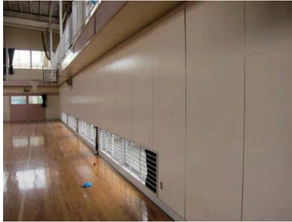
Figure 1.14 2011 Tōhoku ( M_w=9.0 ): temporarily shored damaged interior PW within a gymnasium within the Ibaraki prefecture, Japan. (From NILIM, 2011)
