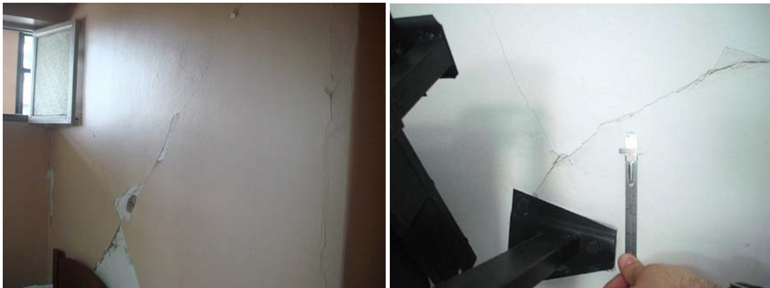
Figure 1.11 2010 Maule (Chile) Earthquake ( M_w = 8.8 ): interior PW damage from Main Santiago Hospital : (a) in-plane damage and (b) damage imposed from attached television monitor. (Photos from G. Pekcan)
