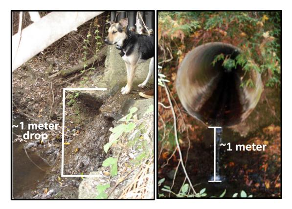
FIGURE 7: Examples of seasonal fish passage barrier due to insufficient water depth in culvert crossing (Site 14)
