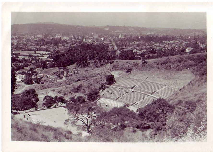
FIGURE 42: WPA Workers Building Will Rogers Bowl, Santa Barbara
