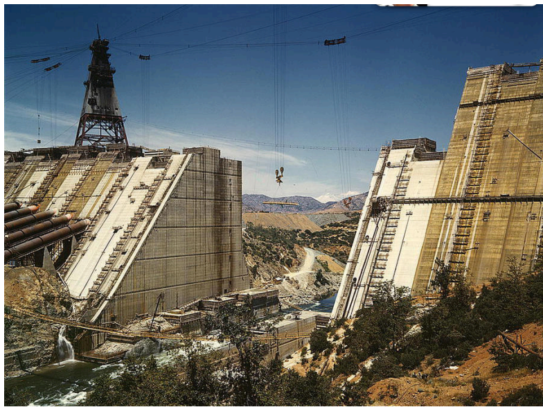
FIGURE 30: Shasta Dam Under Construction, 1939 Built by Bureau of Reclamation
