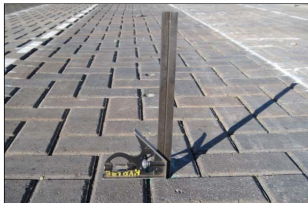
Figure 6.13: Jointing stone depth measurement.
