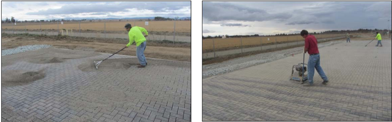
Figure 5.16: Jointing stone placement and compaction.
