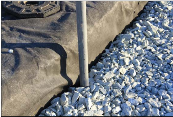
Figure 6.3: Perforated pipe for water level measurements.
