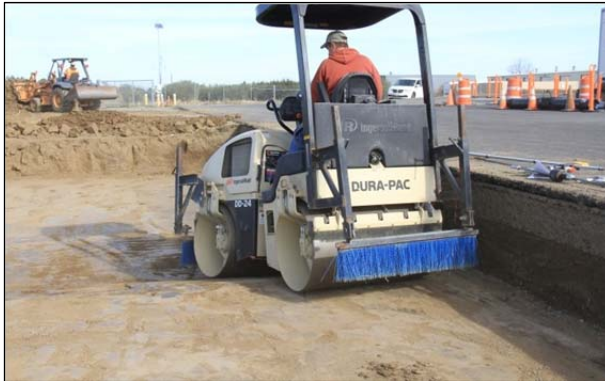
Figure 5.2: Subgrade compaction.
