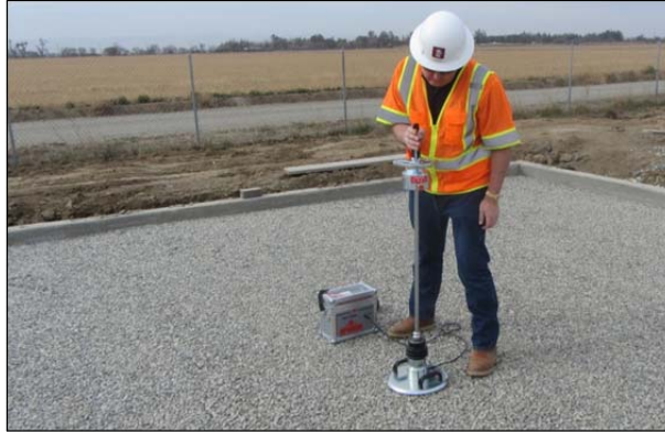
Figure 5.13: Light-weight deflectometer testing on the base.
