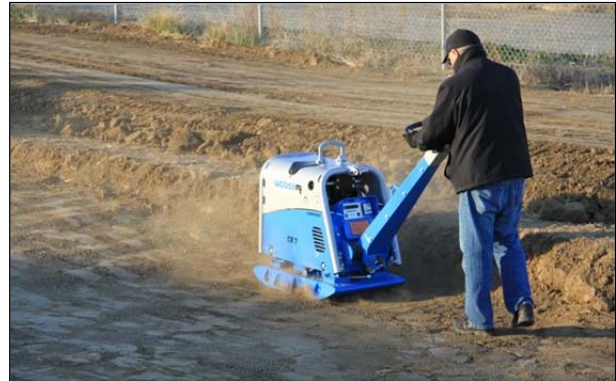
Figure 5.2: Subgrade compaction.
