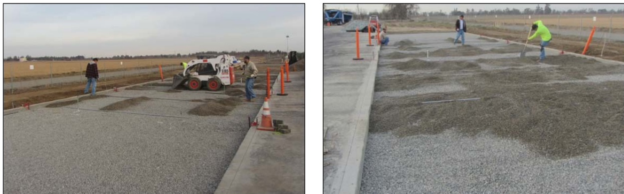
Figure 5.14: Bedding layer placement.
