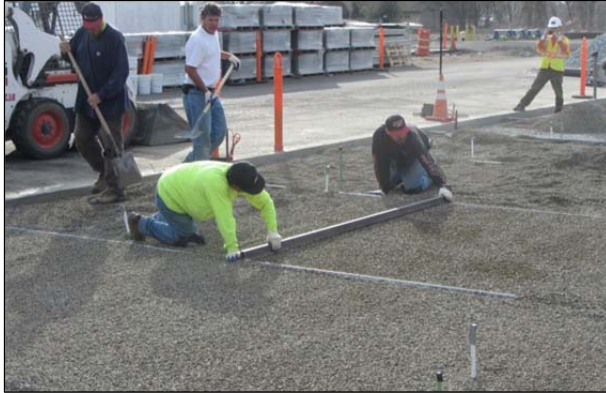
Figure 5.13: Bedding layer placement.
