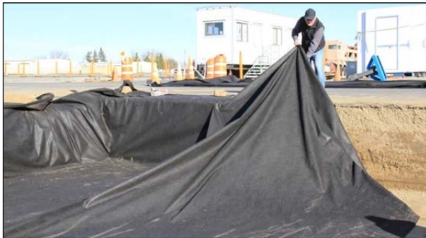
Figure 5.7: Geotextile placement.
