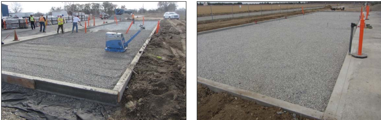
Figure 5.12: Base layer placement.
