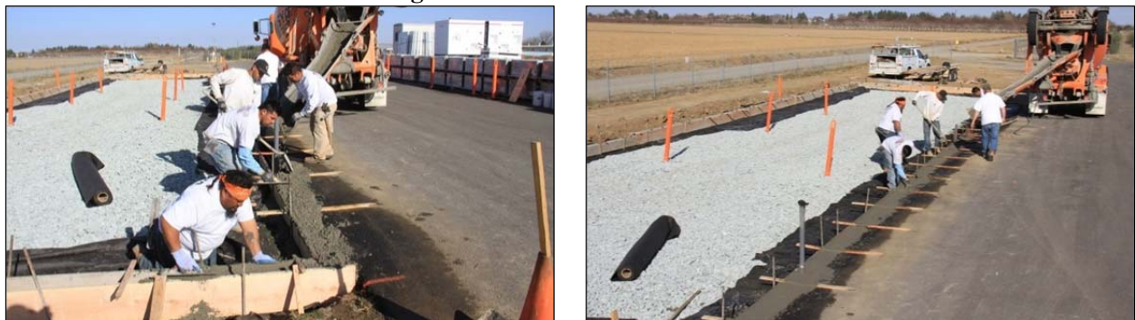
Figure 5.9: Formwork for curb.
