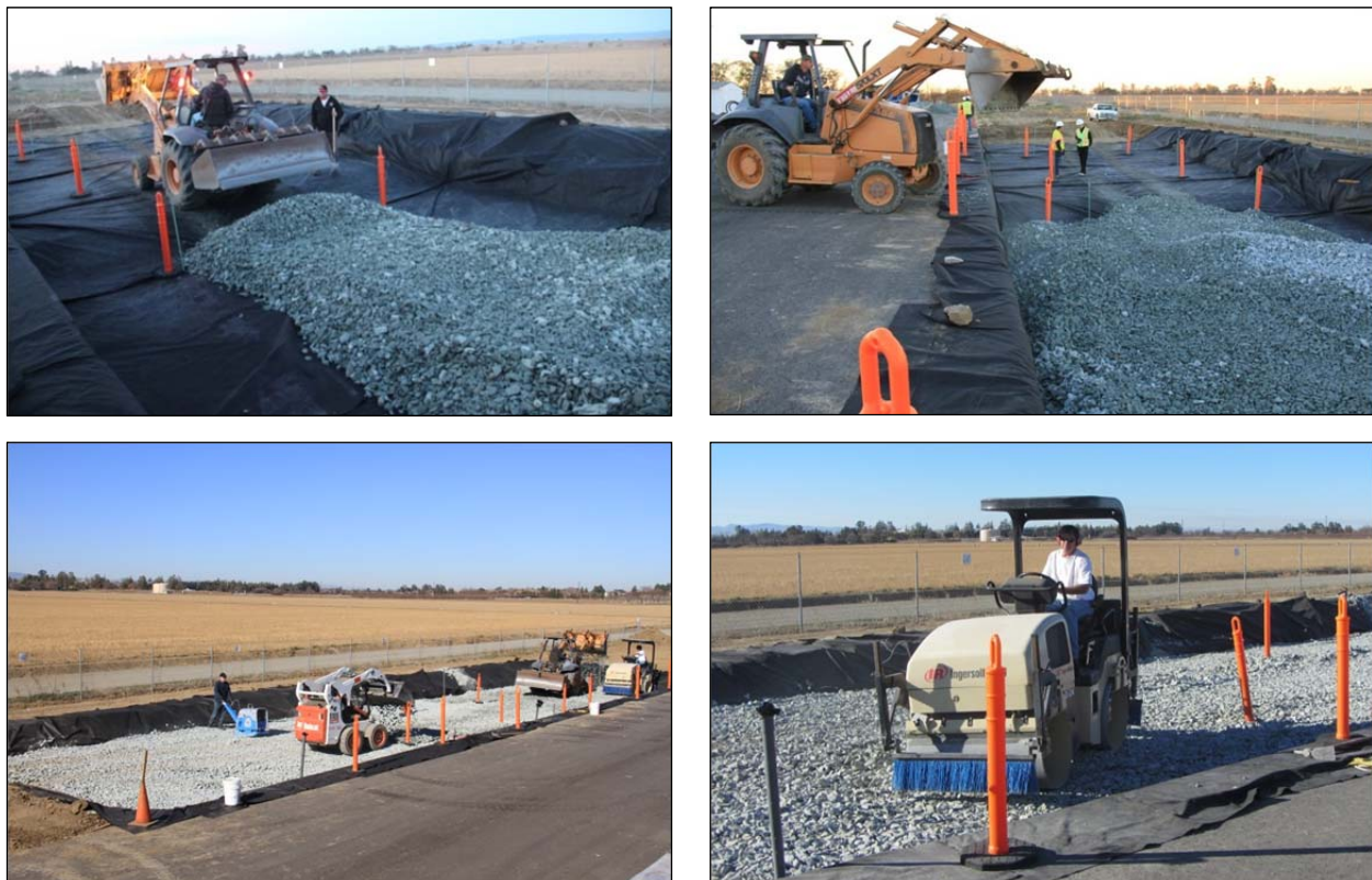
Figure 5.8: Placing and compacting the subbase.
