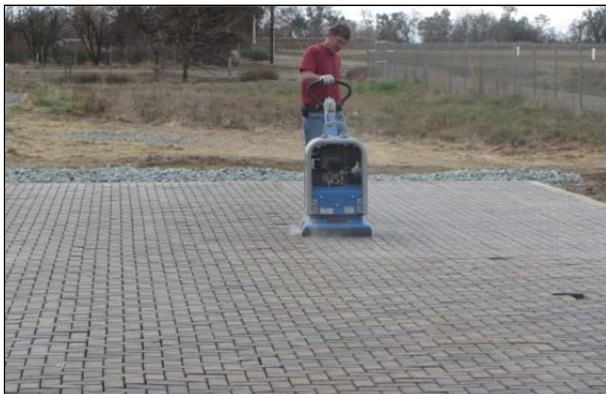
Figure 5.15: Paver placement and compaction.
