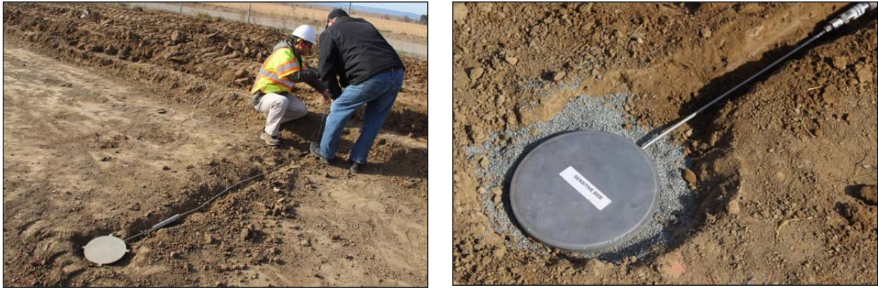
Figure 6.10: Pressure cell installation in the subgrade.
