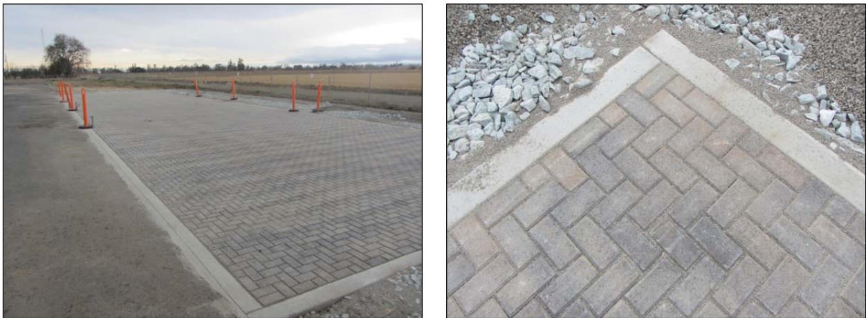
Figure 5.17: Completed test track.
