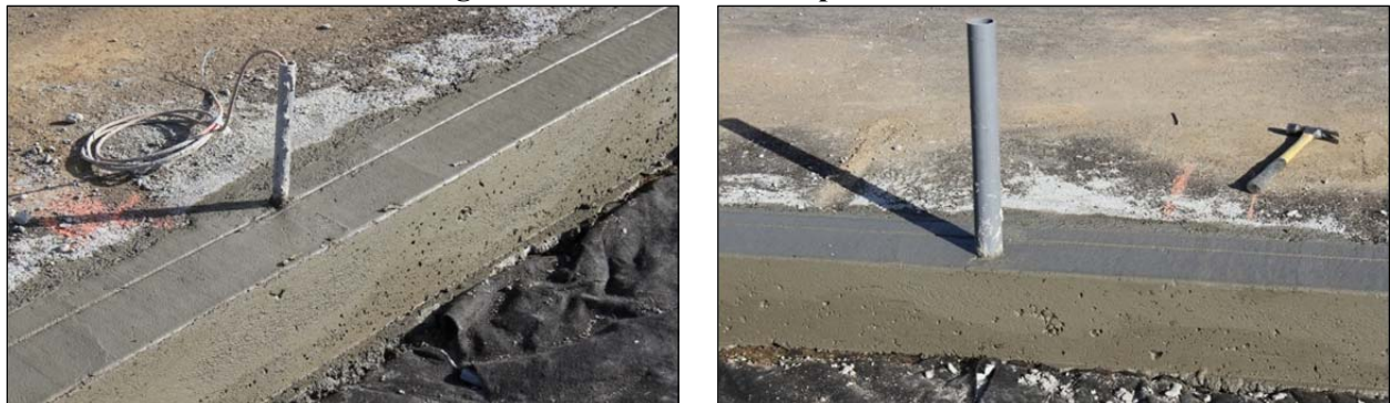
Figure 5.11: Completed curb after removal of formwork (pipes are for instrument wiring).
