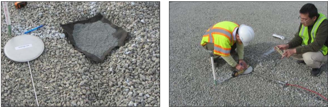
Figure 6.11: Pressure cell installation on top of the subbase.
