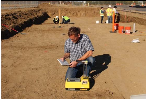
Figure 5.5: Density measurements.
