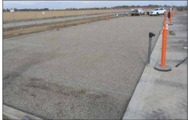
Figure 5.13: Bedding layer placement.
