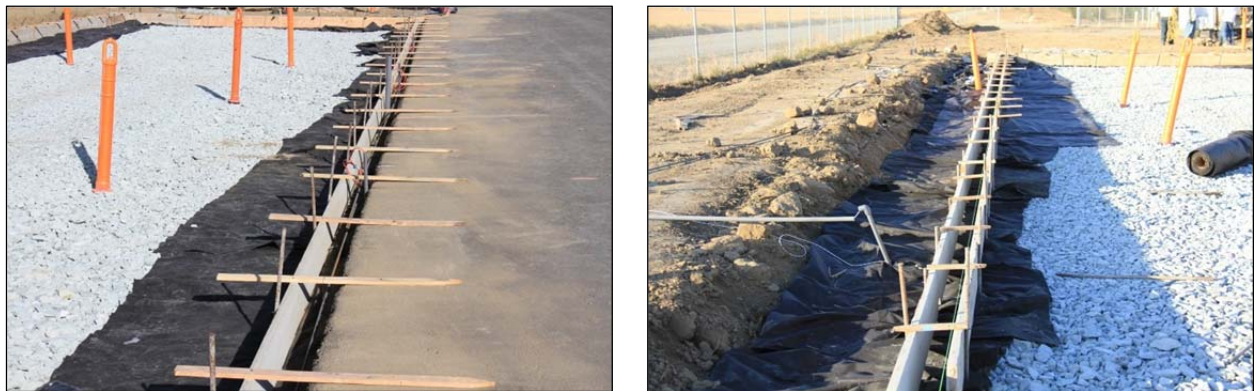
Figure 5.9: Formwork for curb.
