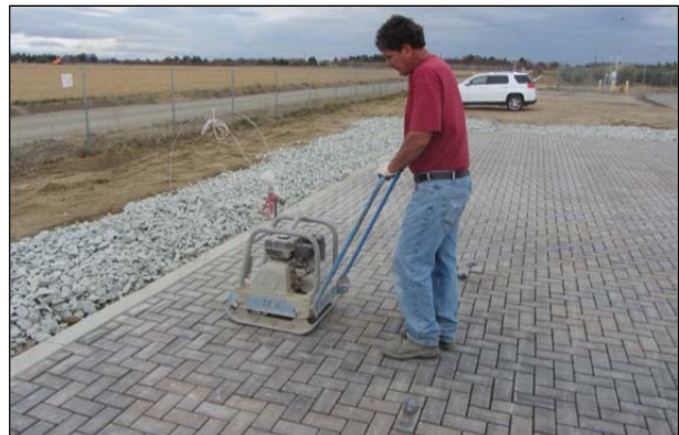
Figure 5.15: Paver placement and compaction.
