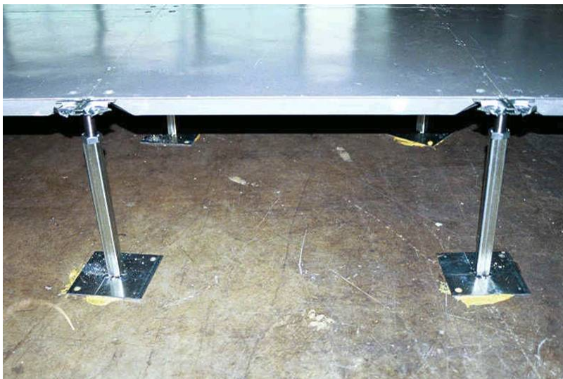
Figure 2-4 Typical Raised Floor Construction
