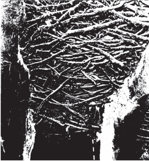
Fig. 3.30 The structural bases of the ceiling on wooden beams and branches. Source: Hirshfeld, 1982.
