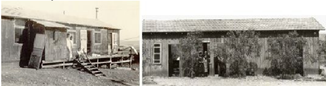
Fig. 5.23 The first ‘rail’ shacks in Beit Alpha did not include porches but a wooden deck to level it with the hilly topography. Each room included a door and two windows on opposite facades for ventilation. In this picture we can see an addition to one of the rooms at the expense of the deck. The original door is leaning against the addition. Source: Beit Alpha archive.
