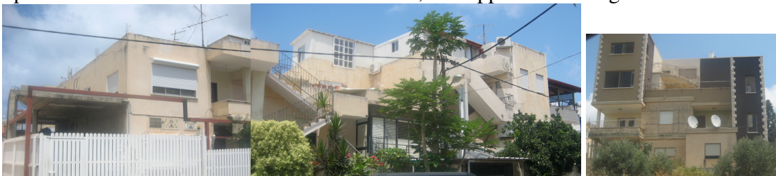
Fig. 7.61 Al-Hassan family house, 2011. Source: Author. Note that the complexity of the house and the fact that it faces a narrow street made it difficult to photograph it from a single spot. This collage is therefore slightly distorted. Fig. 7.62 Apartment houses in Mazraa, 2011. Source: Author.
