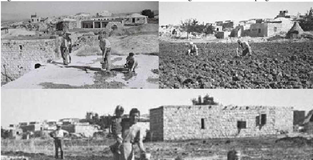
Fig. 6.27, 6.28, 6.29 Moshav Tirat Yehuda, 1949. Source: NPC.
