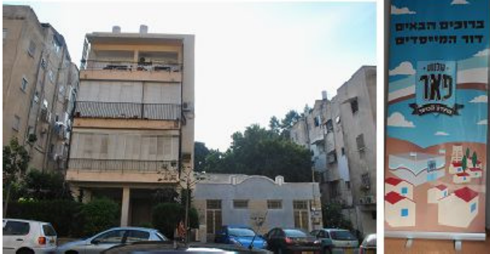
Fig. 4.47 The semi-detached houses on 36 and 38 Yeshayahu street. While house number 36 was torn down for construction of a three storey apartment house in the 1940s, the house on number 38 still stands. Fig. 4.48 A poster welcoming the neighborhood founders to a gym newly opened at the site of the old cinema. Source: Author.
