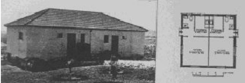
Fig. 6.17 The ‘blockon’ house: two family units of 24 square meters each. Source: Zaslwsky, 1954.
