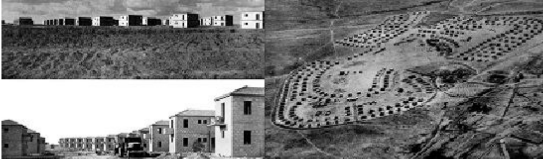
Fig. 6.84, 6.85 First houses of the neighborhood unit in process of construction. Source: Physical Planning in Israel 1948-1953 , Sharon archive.
