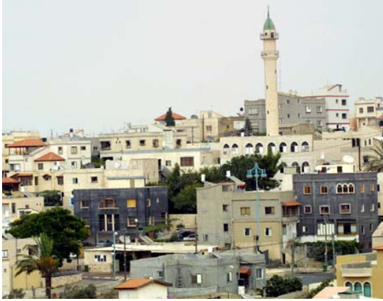
Fig. 0.22. Examples of Sumud housing in the village of Sahnin in the Galilee. Source: Author.
