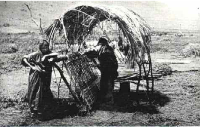
Fig. 3.27 The building of a straw structure for a mud hut. Circa 1900. Source: Zeev Galili archive
