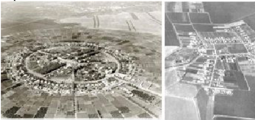
Fig. 8.69 Moshav Ram-On in the Taanach, Jazreel Valley, 1965. Source: Ram-On. Fig. 8.70 Nahalal, 1930s. Source: Bitmuna.
