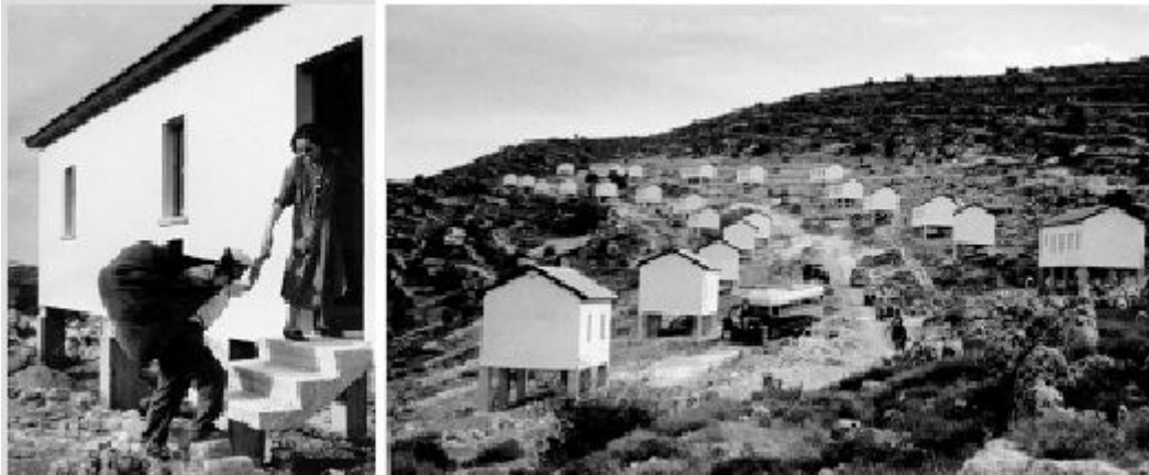
Fig. 6.65, 6.66 First permanent houses in Ksalon, 1952. Source: CZA. Note the 'little boxes' nature of the houses, adapted to the hilly terrain with concrete foundations cast on site. Stairs did not always reach the ground.
