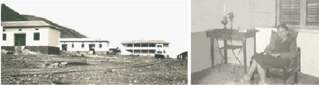
Fig. 5.58, 5.59 The first permanent housing structures in Beit Alpha during construction. The two-storey children's house can be seen in the background. Circa 1930. Source: Beit Alpha archive.
