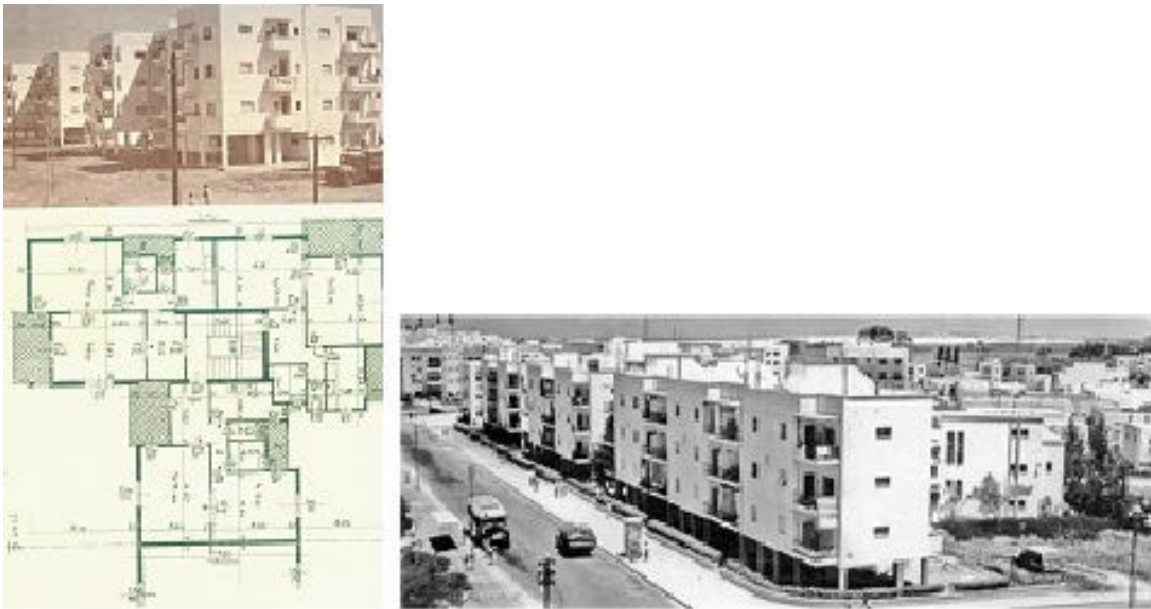
Fig. 4.71 The SELA housing for National Workers on IbnGabirol st. 1952. Source: Jabotinski Institute archive. Fig. 4.72 The RASCO housing complex on Milano square built for the Jewish Agency, housing white collar workers and ‘the middle class’. Design by Lotte Cohn. Source: Sonder, 2010.
