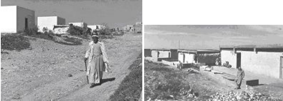
Fig. 7.22 New housing built in the village of Makr, near Acre, March 1950. At the back are the old houses of Makr. Photographer: Fritz Cohen. Source: NPC.
