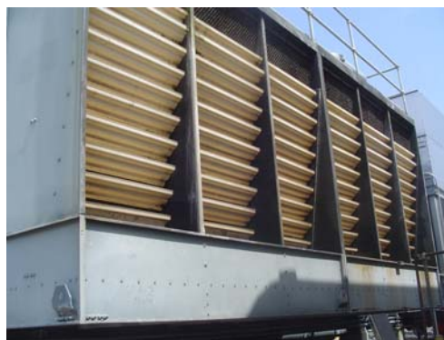
Figure 9. cooling tower for chillers at the San Diego P&DC
