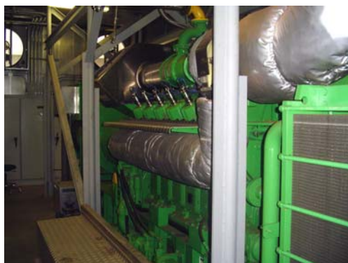
Figure 8. General Electric Jenbacher 1.5 MW reciprocating engine installed at the San Diego P&DC
