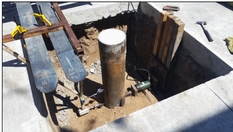
Figure 4.77: Lateral load testing set up for pile test 1 at LAX
