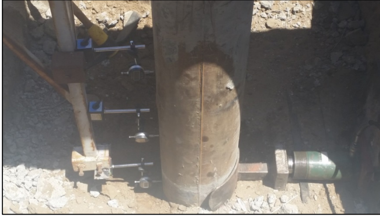
Figure 4.78: Lateral load testing set up for pile test 1 at LAX
