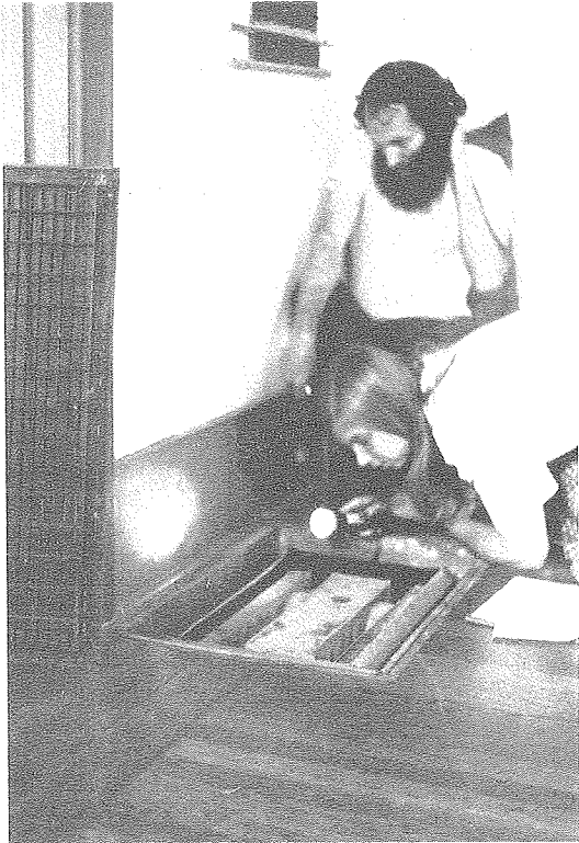
Fig. 1. Many Berkeley homes are heated with gas floor furnaces, which when they are not in operation (most of the time) are sources of considerable quantities of cold outside air. (XBB 783-3191)
