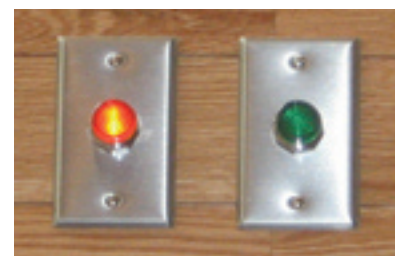
Signals are installed at either end of each floor in public circulation areas.
