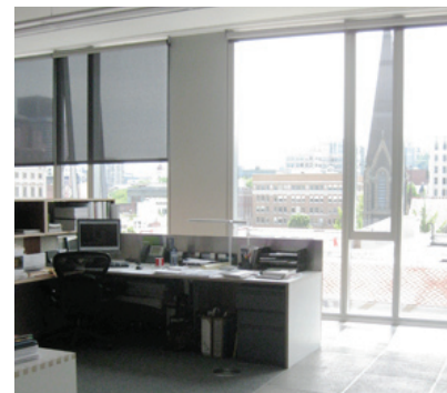
Operable slender awning windows are removed a few feet from workstation clusters
