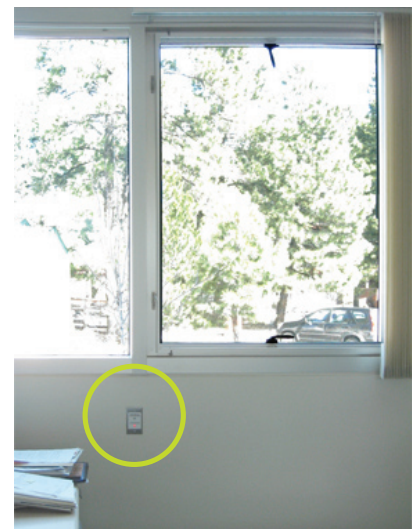
Signals are located below the window in each private office
