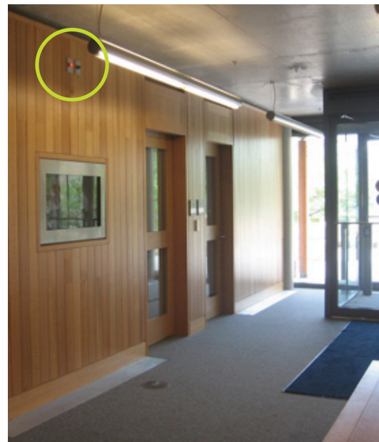
Signals are installed at either end of each floor in public circulation areas.
