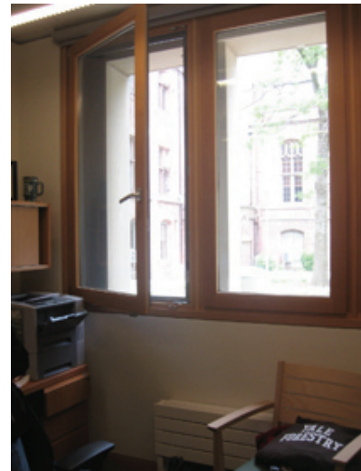
Typical office "tilt-turn" window
