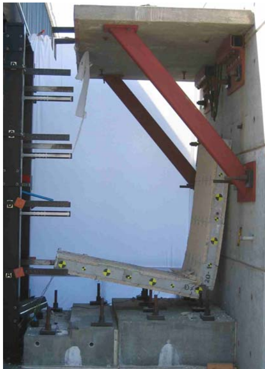
Figure 5.20: Series I Test 5- Post test damage
