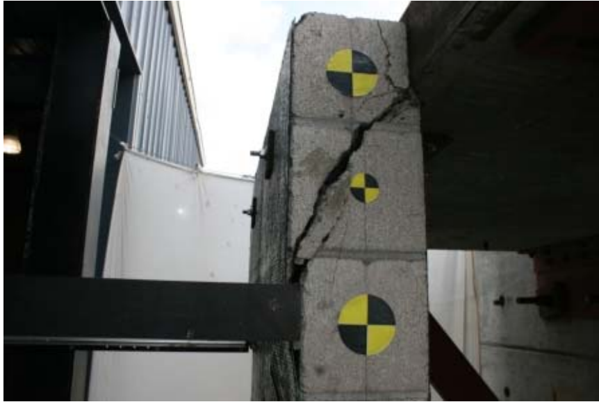
Figure 4.32: Test 6- CMU 3 damage at top
