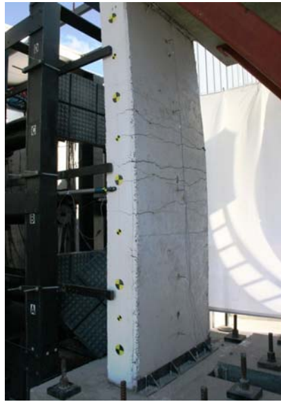
Figure 5.44: Series II 12 in. RC wall, typical damage
