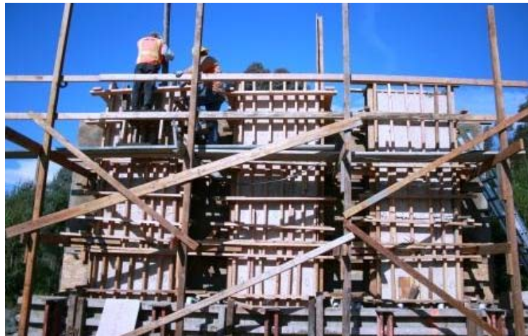
Figure 5.30: Bracing of frangible panels following blow out
