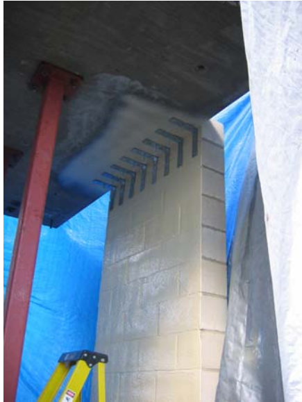
Figure 6.8: Angles attached to support over first layer of polyurea
