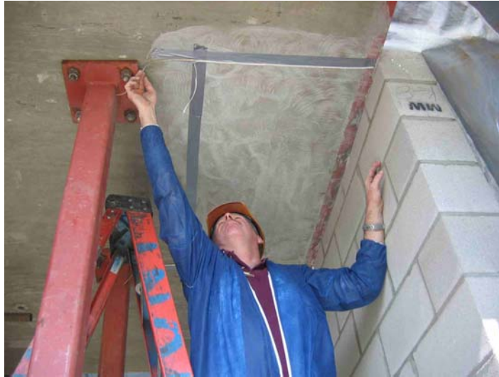
Figure 6.4: Wire tape before surface polyurea applied
