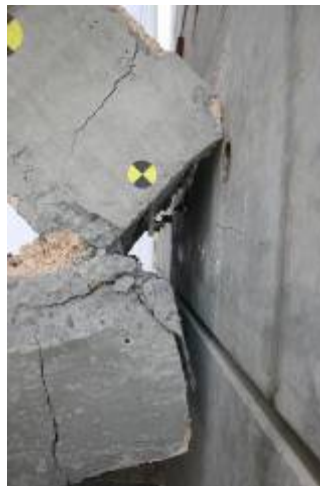
Figure 5.42: Series II Test 2 midspan failure
