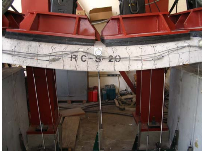
Figure 5.14: Series I Static Test 1- RC-S-20 wall cracks
