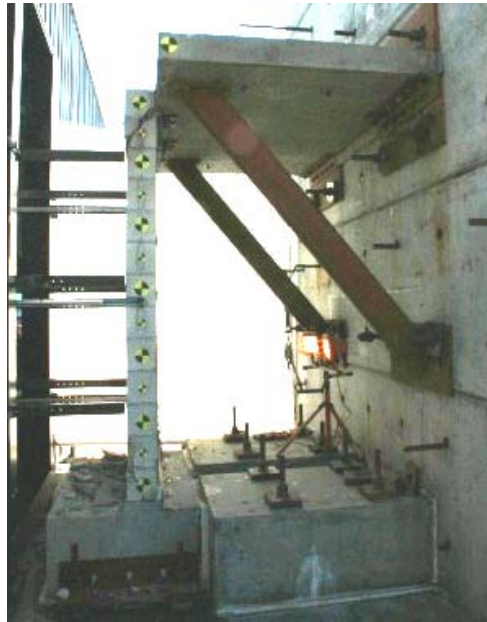
Figure 4.17: Test 3- CMU 1 post test
