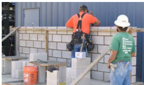
Figure 3.22: CMU wall construction
