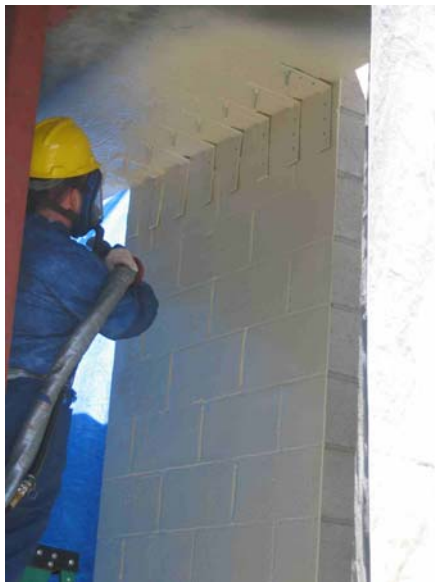
Figure 6.9: Angles coated with second layer of polyurea
