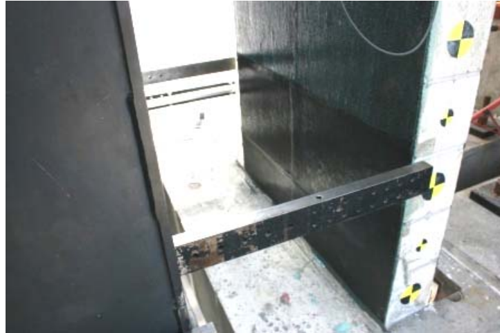
Figure 4.27: Test 6- CMU 3 repaired portion of the wall
