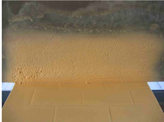
Figure 6.12: Top connection for polyurea with primer
