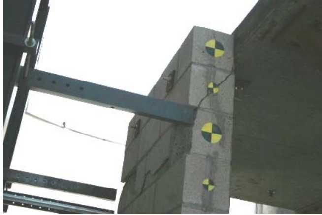
Figure 4.22: Test 4- CMU 2 damage at top
