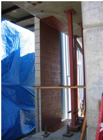
Figure 6.11: XPM Urethane Primer before polyurea application
