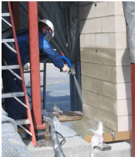
Figure 6.2: Application of polyurea
