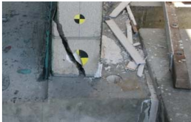
Figure 4.24: Test 5- CMU 3 damage at bottom
