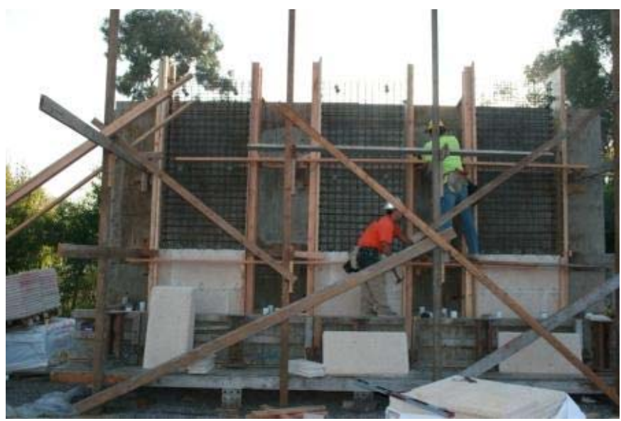
Figure 5.28: Bracing, bulkheads, and scaffolding for frangible panel specimens
