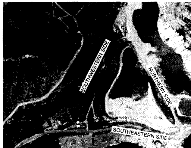
FIG. 2. Aerial Photograph of Pond No. 6 in Tapo Canyon before Northridge Earthquake (Photo by I.K. Curtis, Inc., April 1993)
