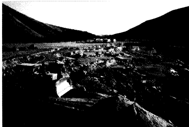
FIG. 8. Photograph of Displaced Concrete Blocks on Surface of Tailings (Note: Trucks in Background for Scale)
